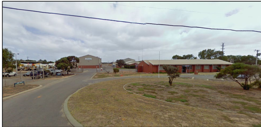
Figure 3: 2010 view of 351 (Lot 277) Eighth Street, Woorree illustrating Oracle Energy depot and office operations (source Google)
