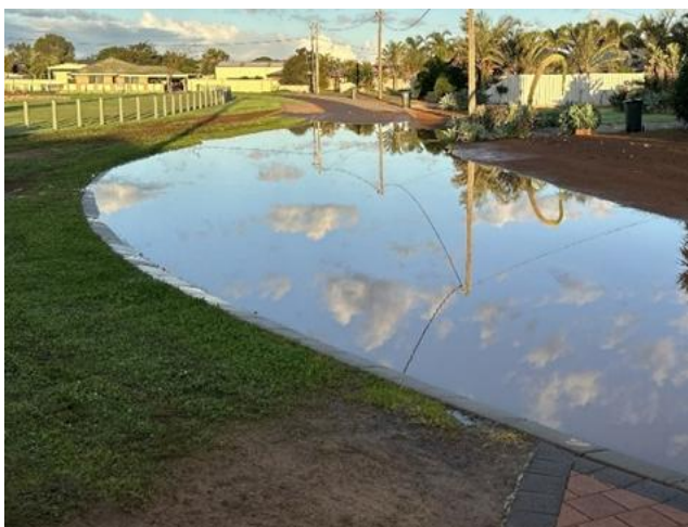
Casuarina Close Sump & Drainage Upgrades
