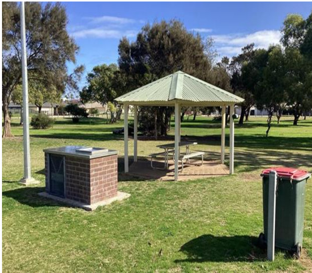
Bayside Park Gazebo Hardstand Renewal
