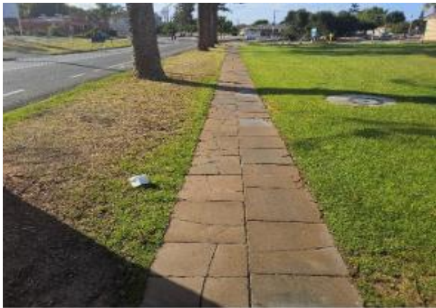
Durlacher Street Footpath Renewal
