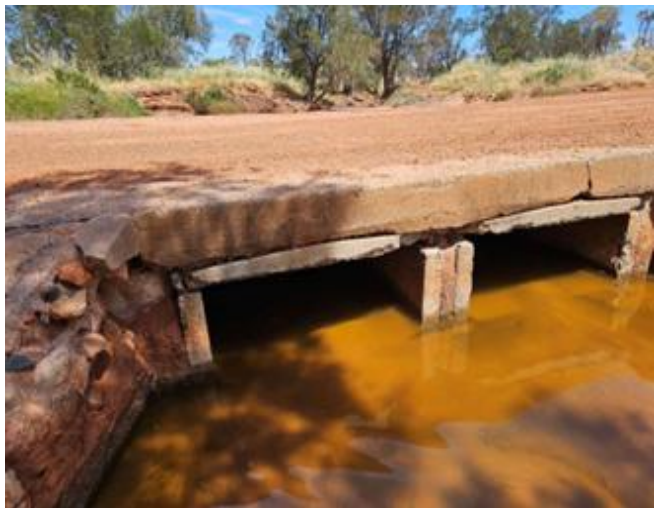
Wongoondy - Tardun Road Culvert Replacement
