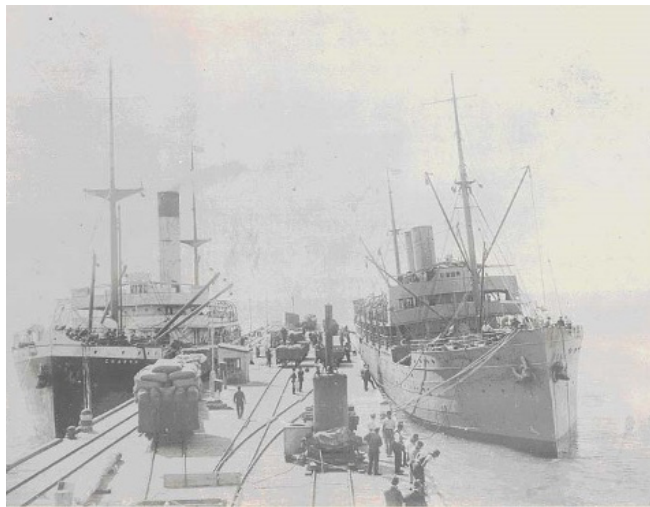
Figure 4 – Geraldton Port, 1920s (Source: Mid West Ports Authority)
