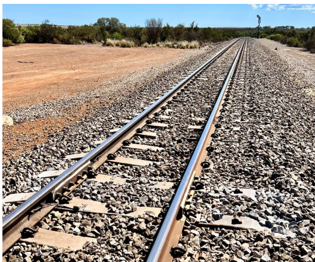
Figure 15 – Gauge Upgradeable Concrete Sleepers (Geraldton-Mullewa Railway)
