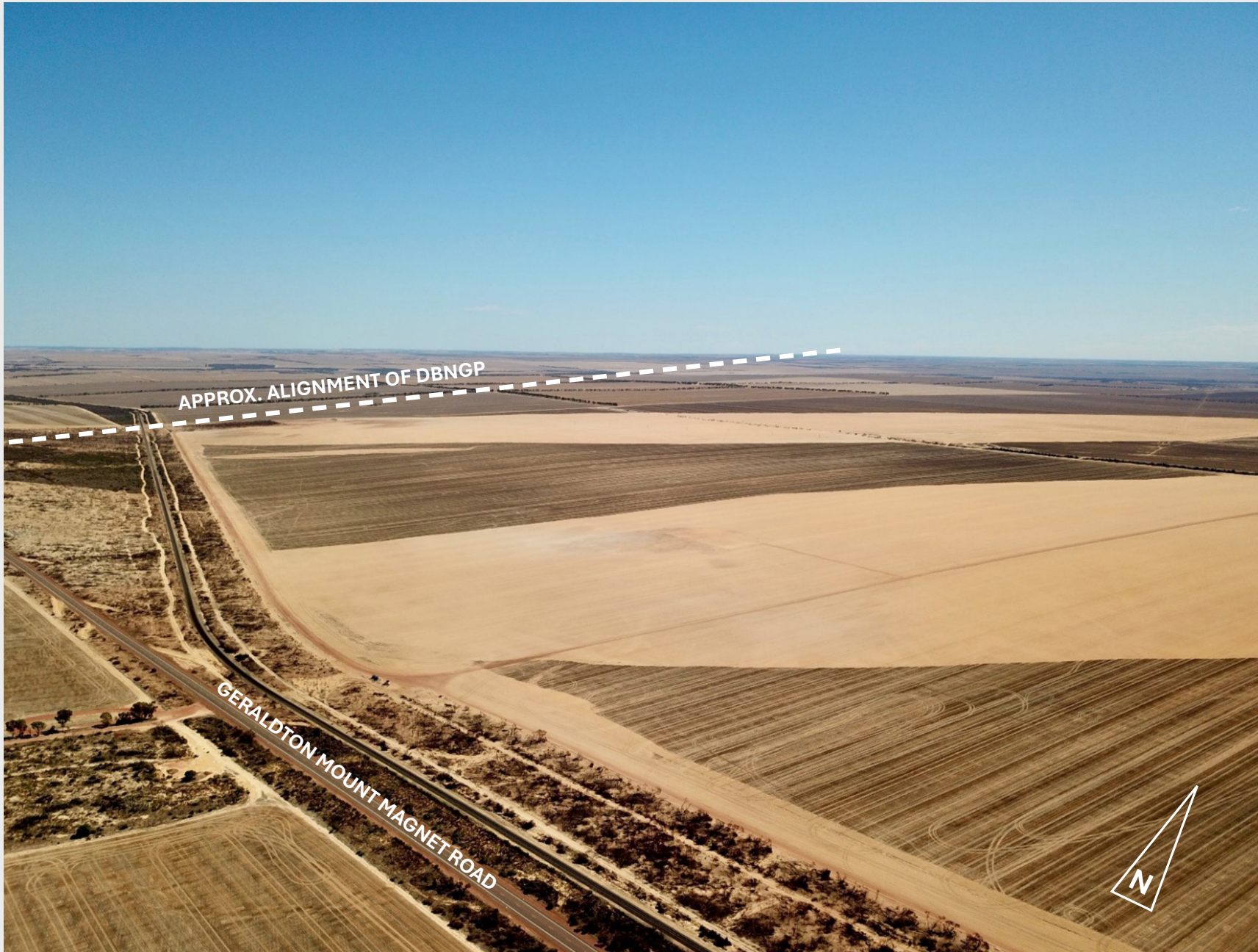
Figure 14 – Drone Imagery of IA 6 showing approximate alignment of DBNGP
