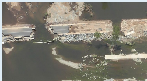
Hillside - Marble Bar Road (severe washout)
