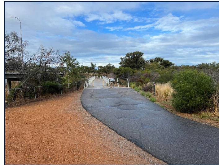
Figure 6 Existing dual use path to pedestrian bridge over Chapman River
