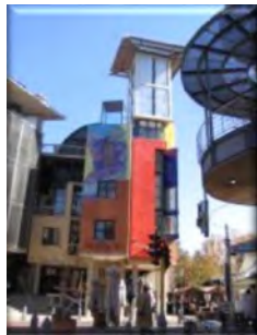
Landmark buildings add character and richness to a city – Moyo development (Johannesburg, South Africa).
