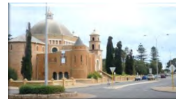
Developments towards the centre of town on Cathedral Avenue should reference and compliment the Cathedral and street trees.
