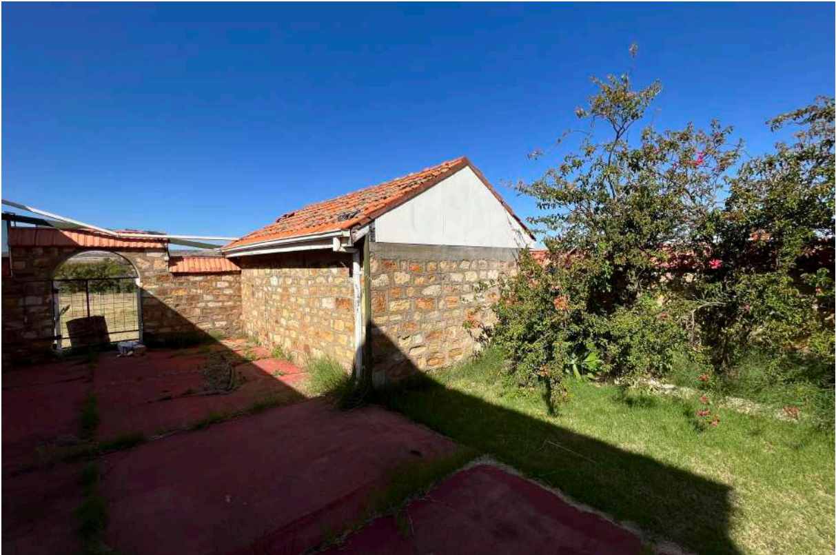
16 North east detached stone store room
