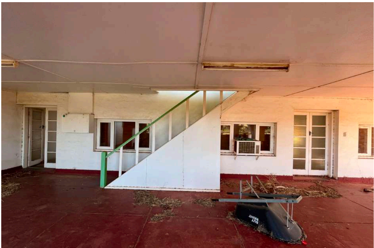
22 External stairs to first floor verandah
