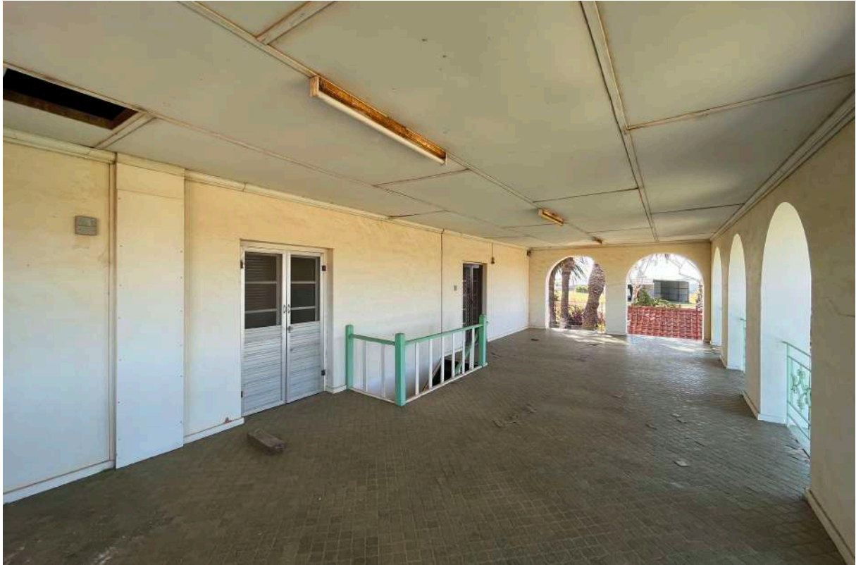
59 First floor balcony
