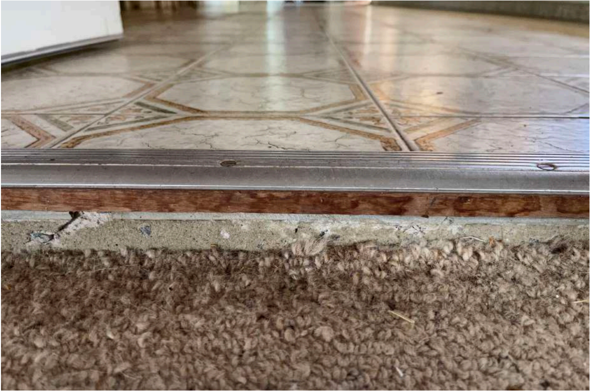
27 Concrete floor overlay to enclosed verandah
