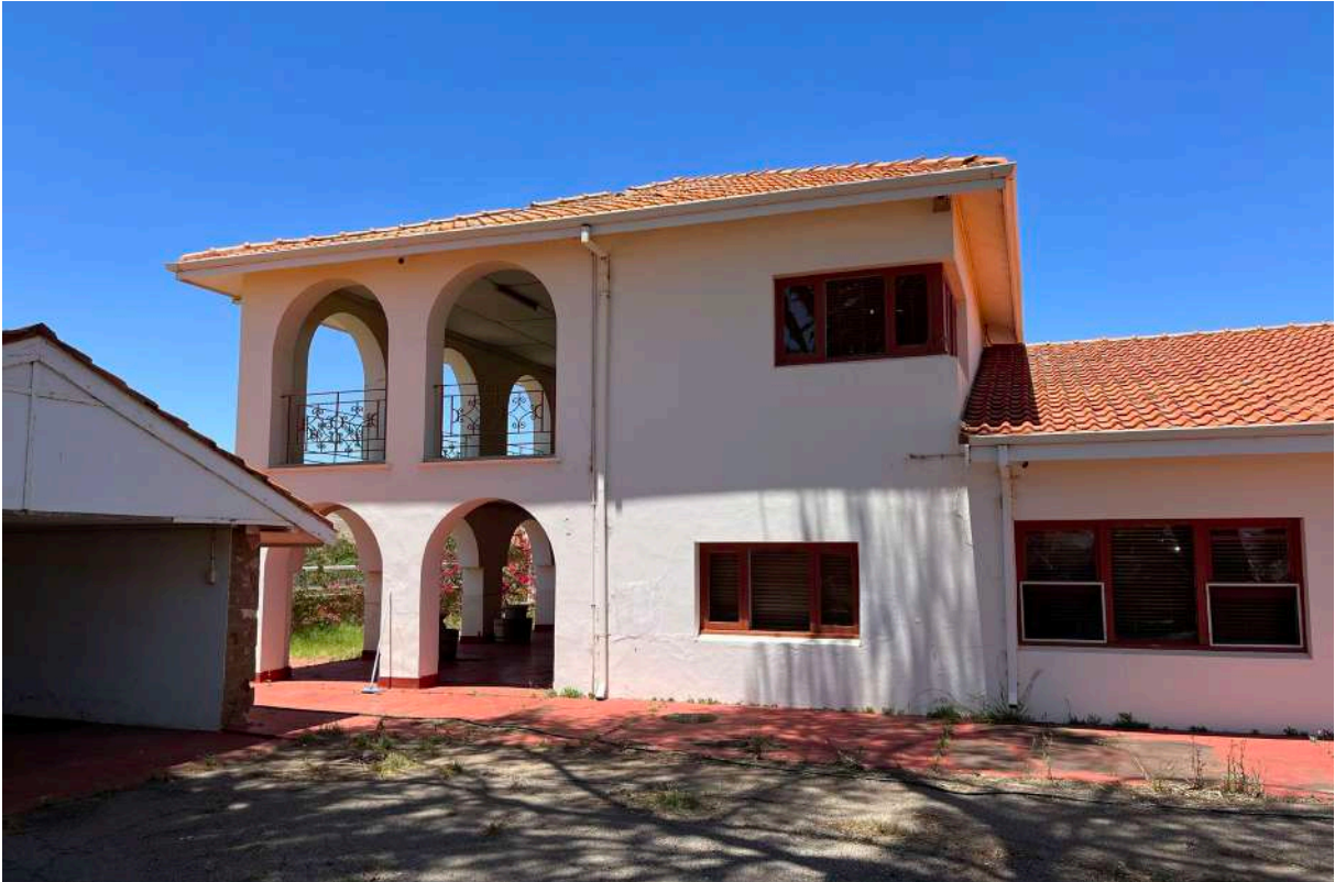
19 West facade of two storey section
