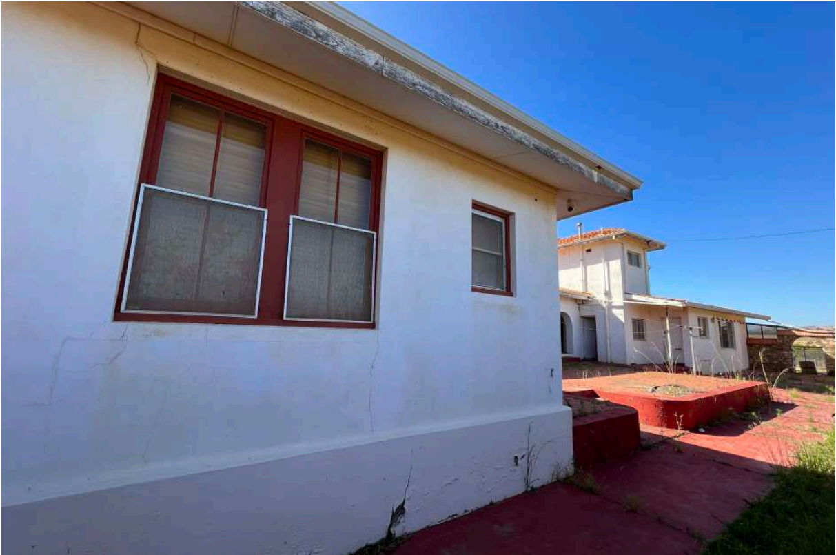
12 South east corner
