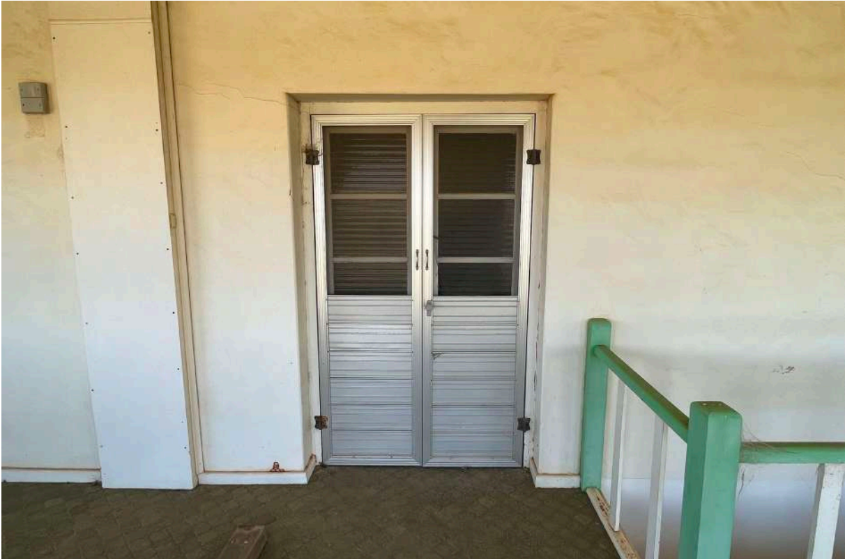
63 Door to first floor robe
