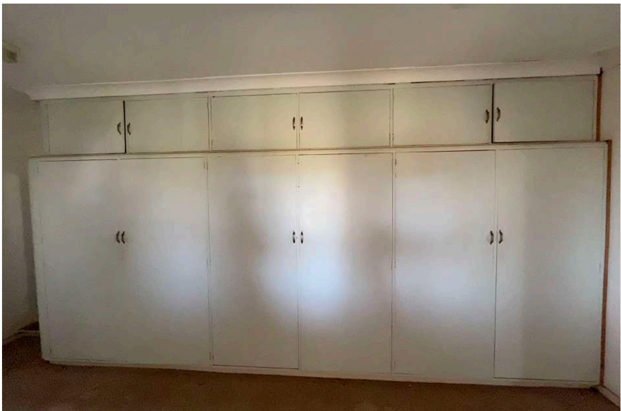
68 Built in wardrobe to first floor
