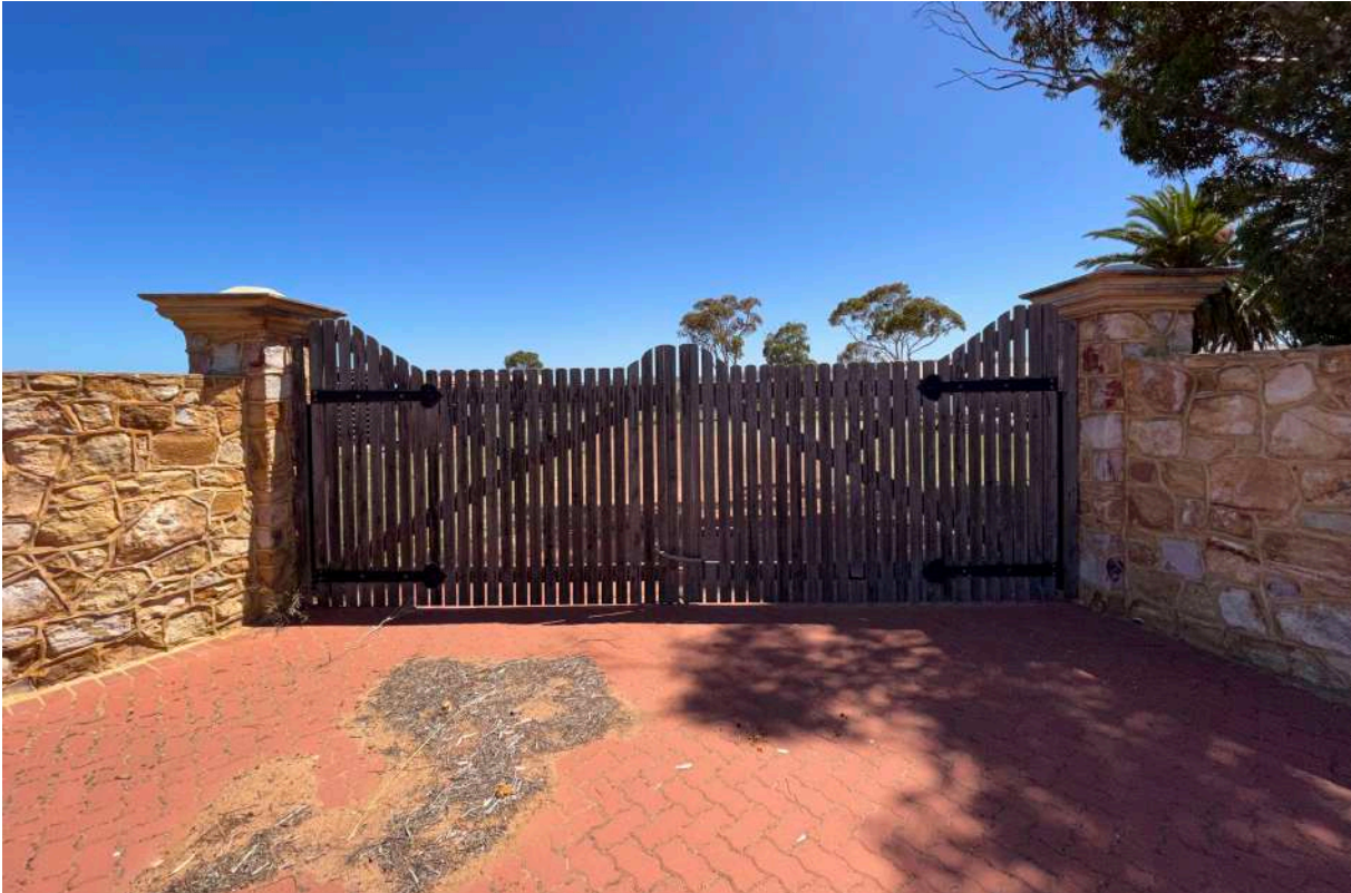
03 Timber entry gate
