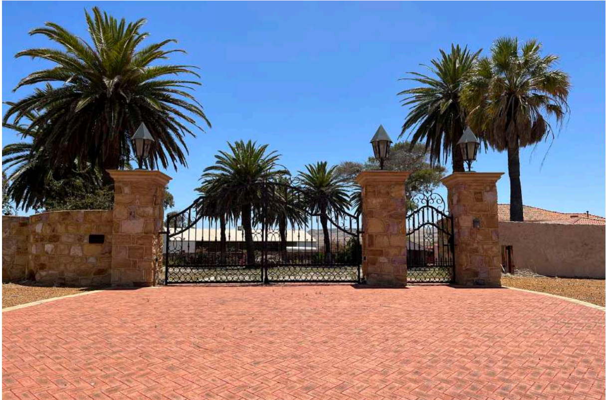
01 Steel Entry Gates
