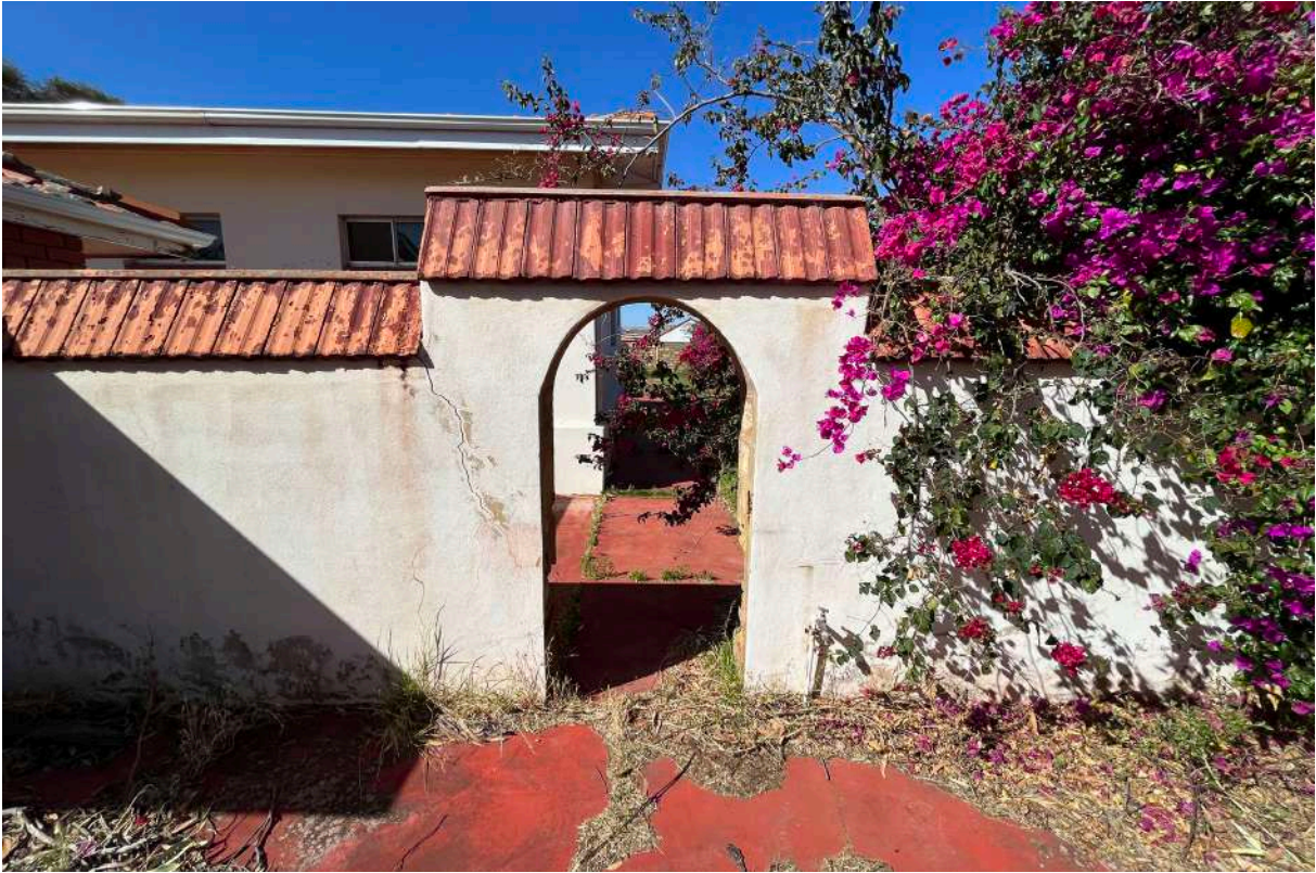
79 Rendered stone wall between Homestead and Workers Accommodation
