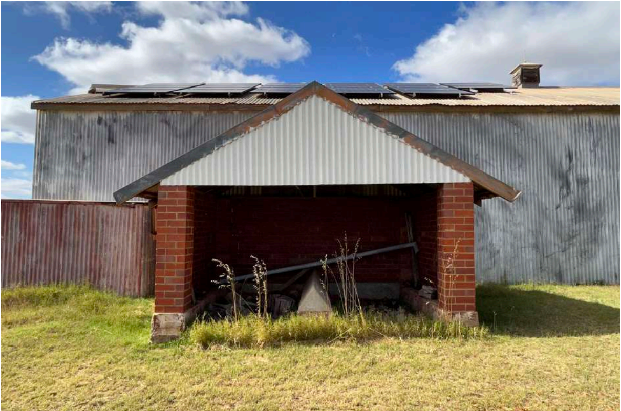
74 Small brick stable to north of Shed 1
