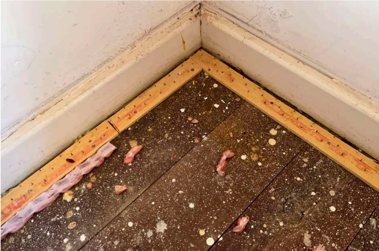
37 Timber floors under carpet to Living 3
