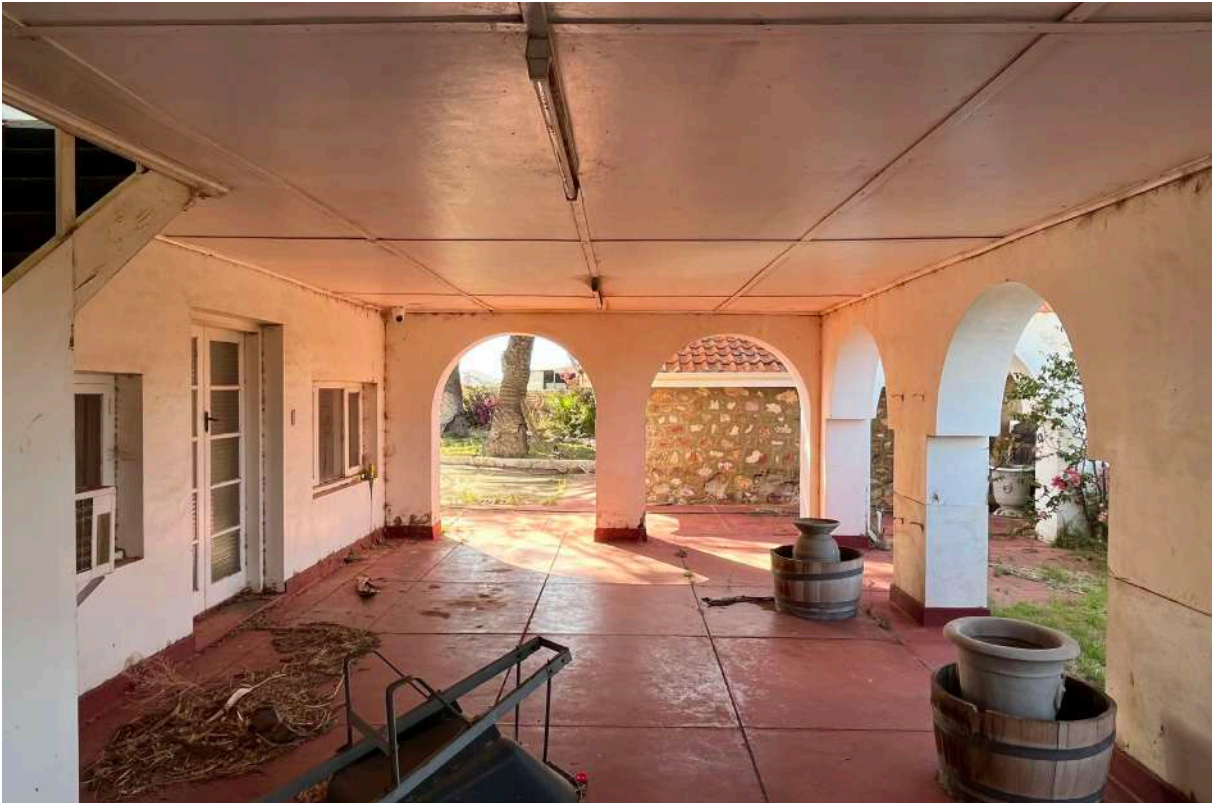
20 Ground floor northern verandah
