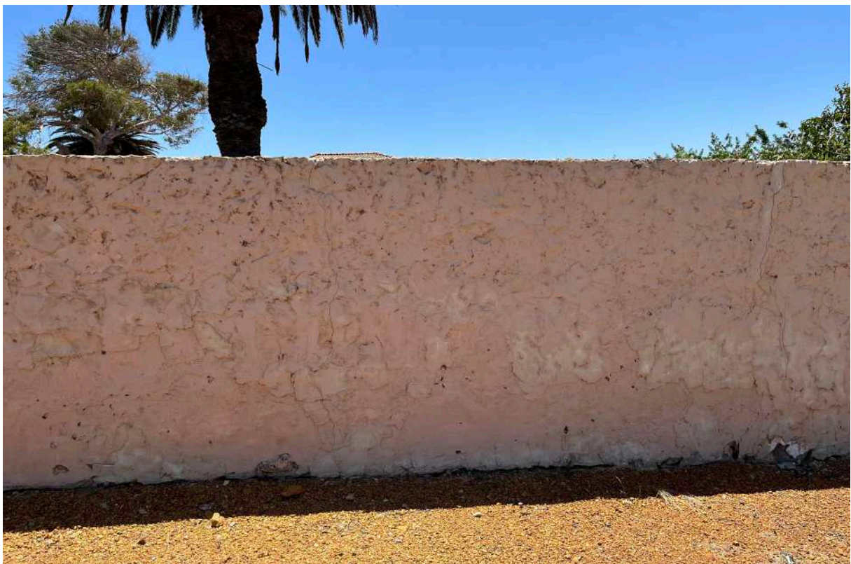
02 Rendered stone perimeter wall
