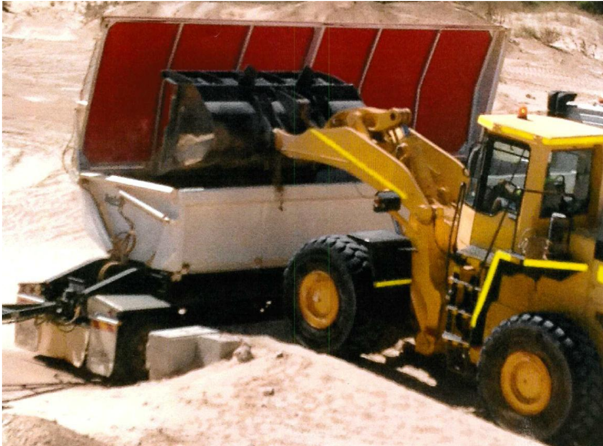
Figure 3.6 Loading Sand Directly into Waiting Road Trucks
