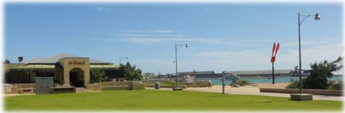
Dome – Geraldton Foreshore
