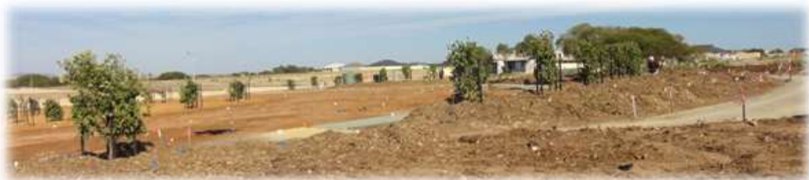
Wanderer Park (under construction) – Wandina
