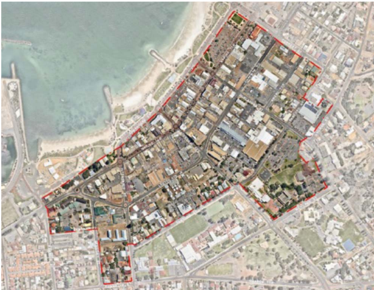
Figure 8: City Centre Revitalisation Project Area
