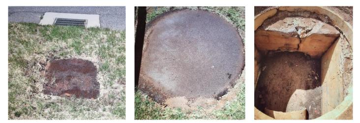
Drainage Renewals example (L-R): Corroded Manhole covers in the verge and cracked pit wall.
