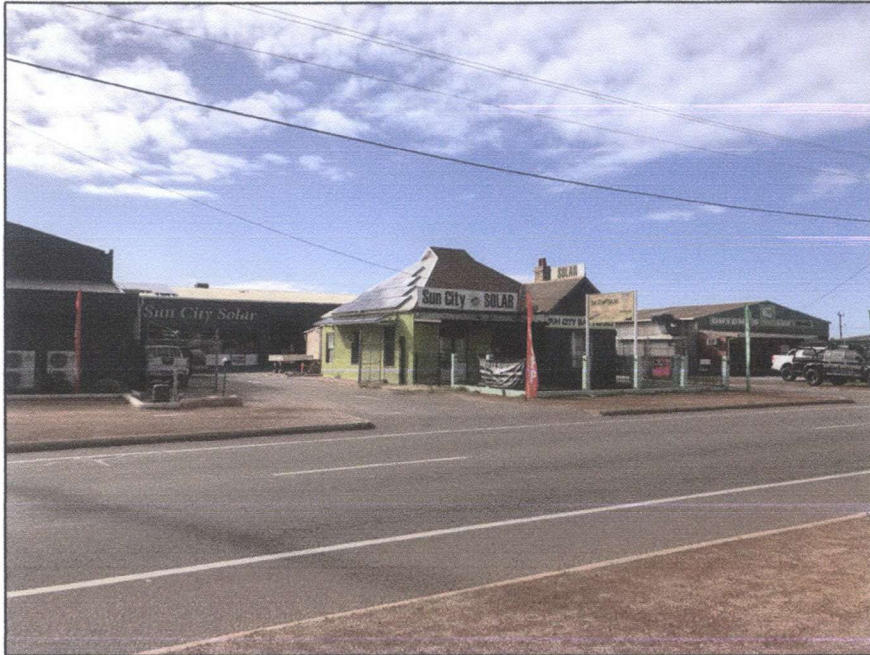
Figure 1 – View of building from western side of Flores Road
