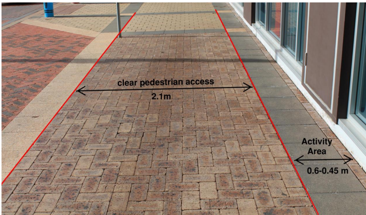
Figure 2 – Marine Terrace from Forrest Street to Durlacher Street. Designated clear pedestrian access location and width and subsequent area available for approval.
