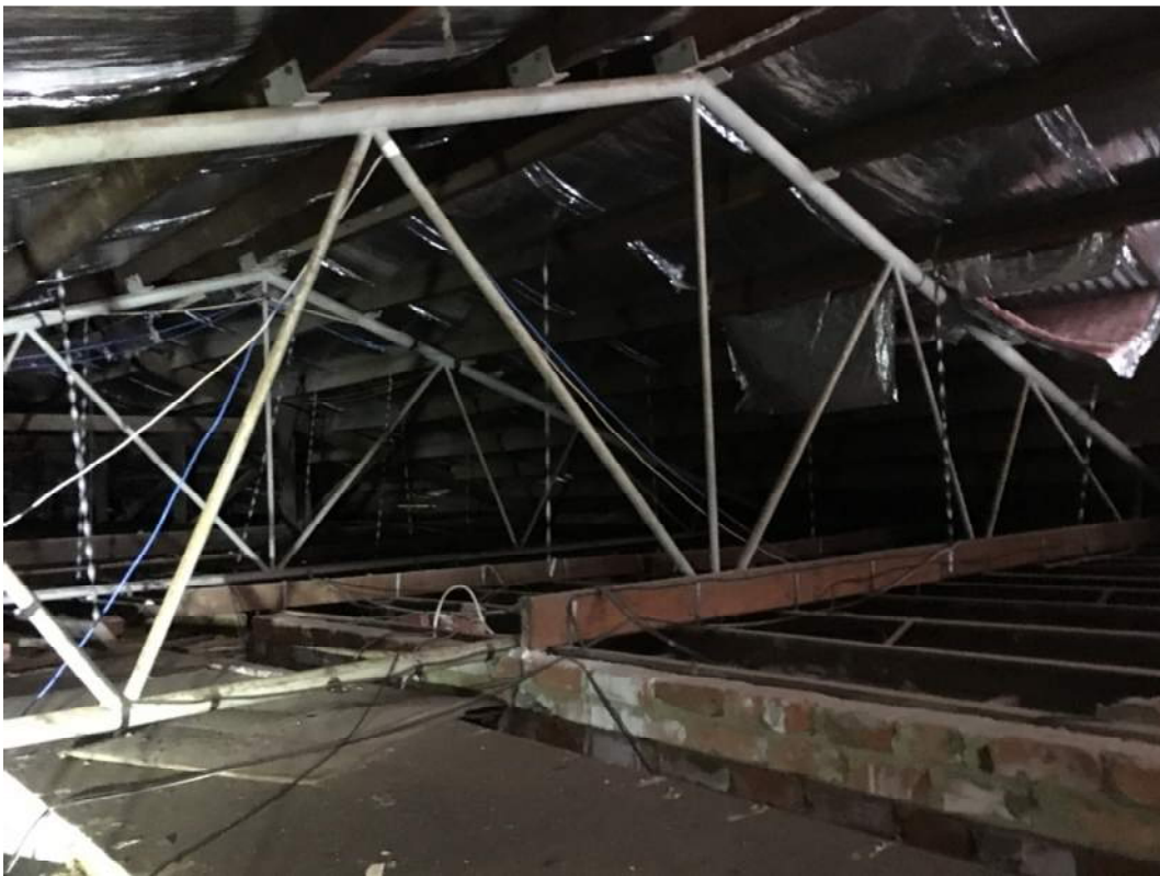
Figure 23: Closeout of steel truss
