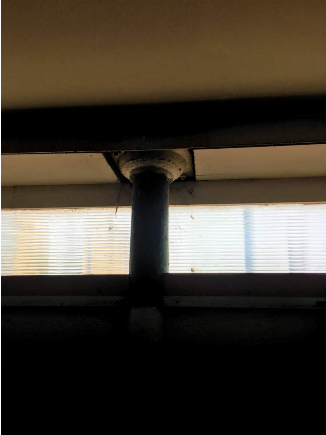
Figure 17: Column head supporting shop front
