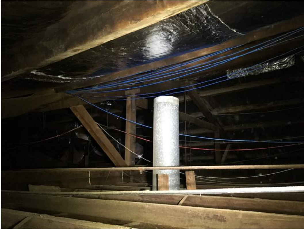
Figure 18: Overall view of timber roof truss
