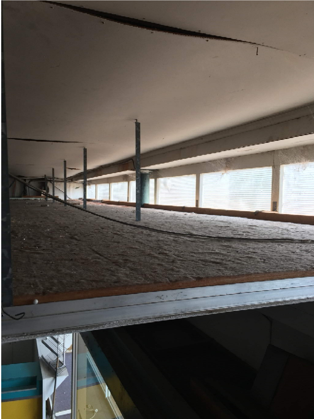
Figure 16: Shop front between plasterboard ceiling and tin ceiling
