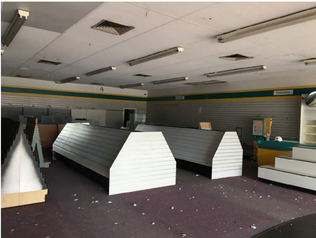
Figure 5: View of front space of building looking north
