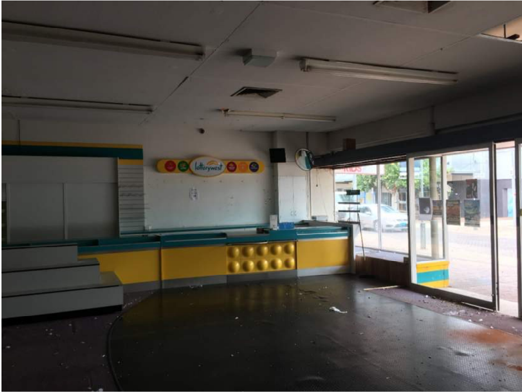
Figure 4: View of front space of building looking east
