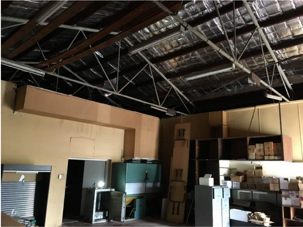
Figure 10: View of rear space of building looking south
