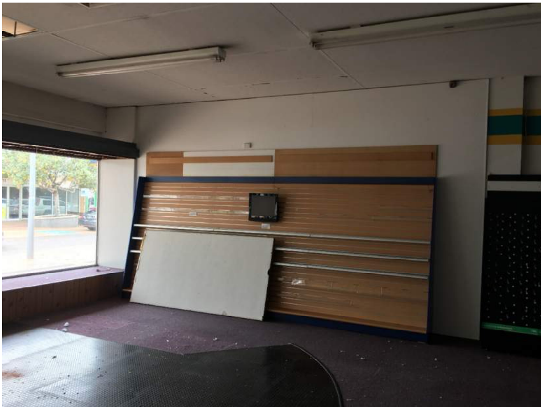
Figure 3: View of front space of building looking south
