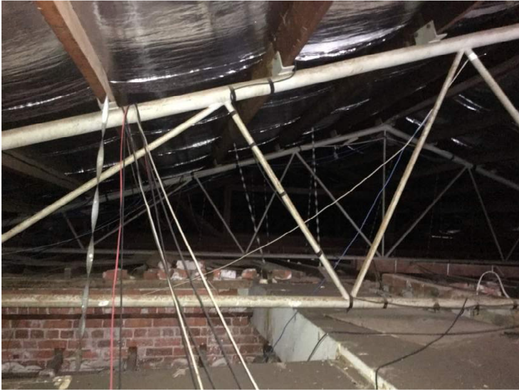
Figure 22: Closeout of steel truss
