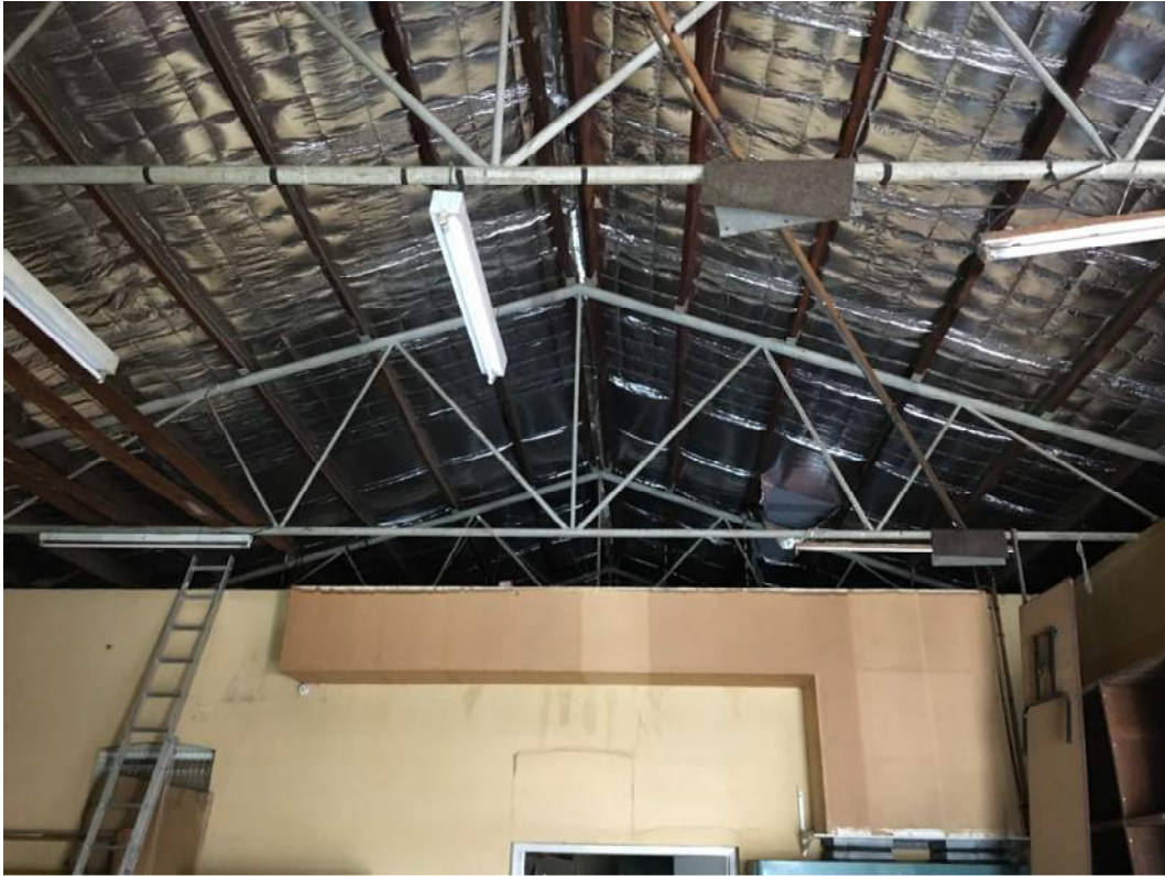
Figure 20: Steel truss from ground level
