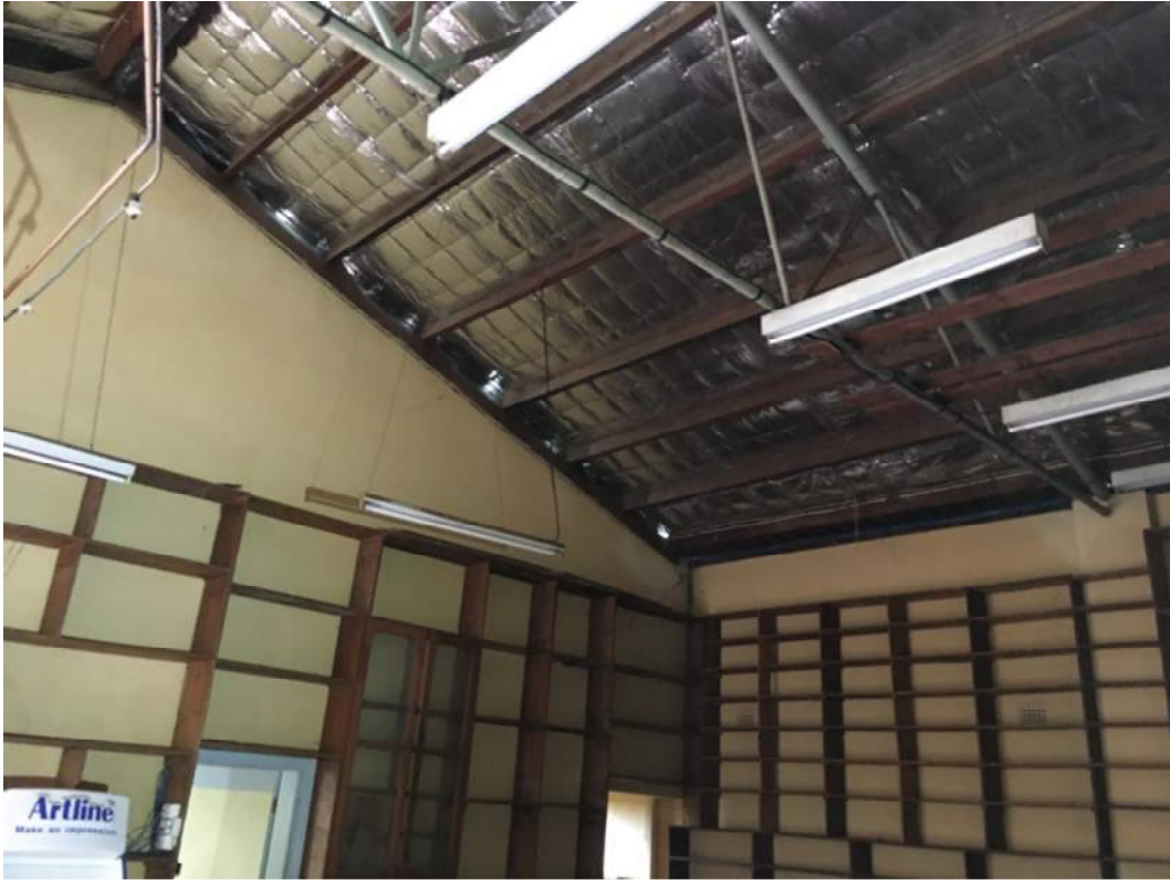
Figure 12: View of rear space of building looking north
