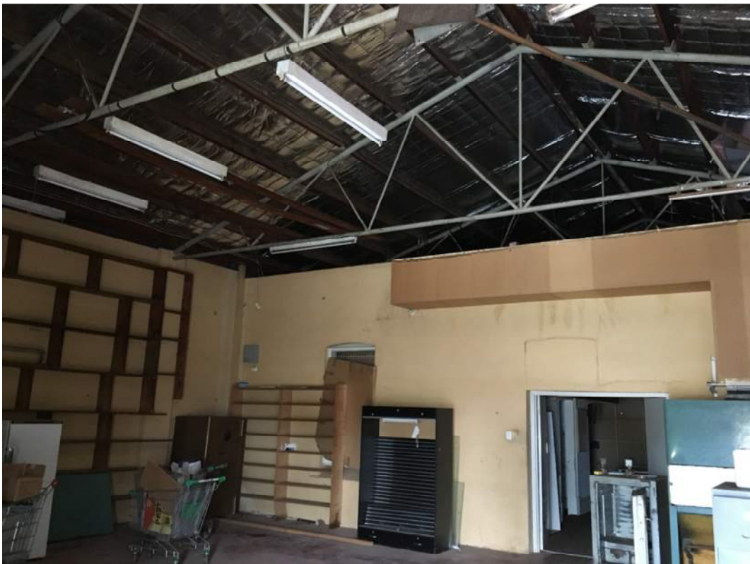
Figure 11: View of rear space of building looking east
