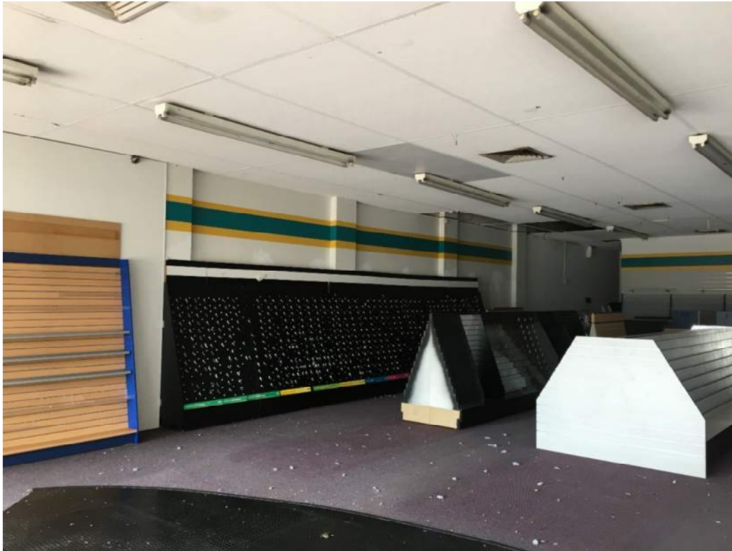
Figure 2: View of front space of building looking west
