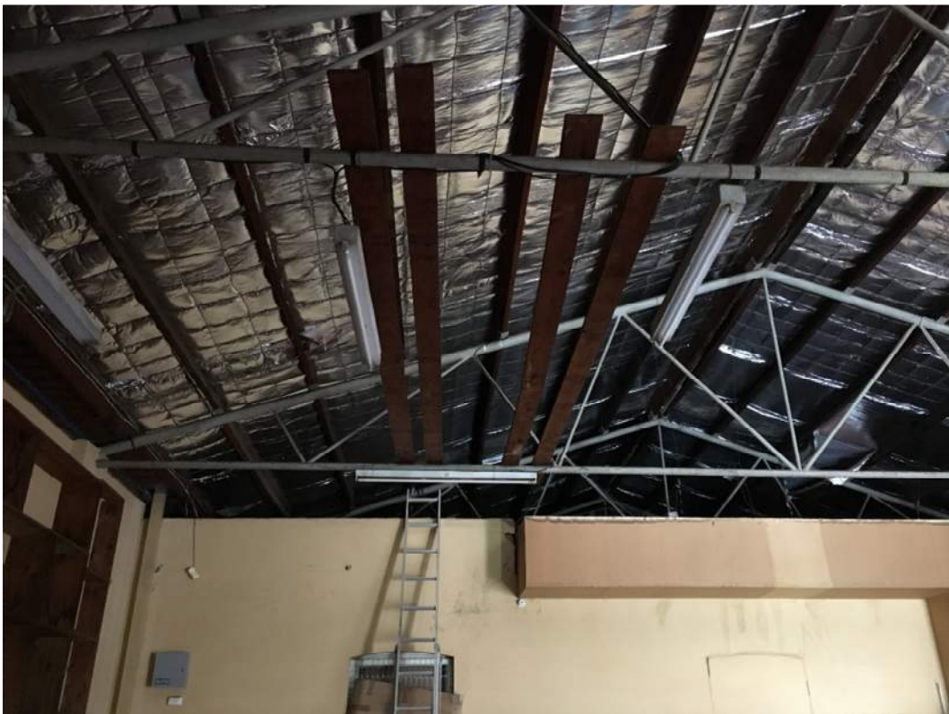
Figure 21: Steel truss from ground level
