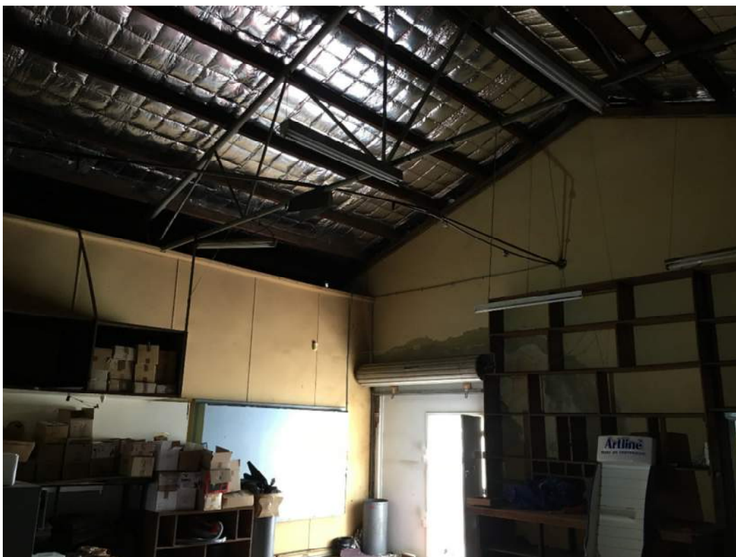
Figure 9: View of rear space of building looking west
