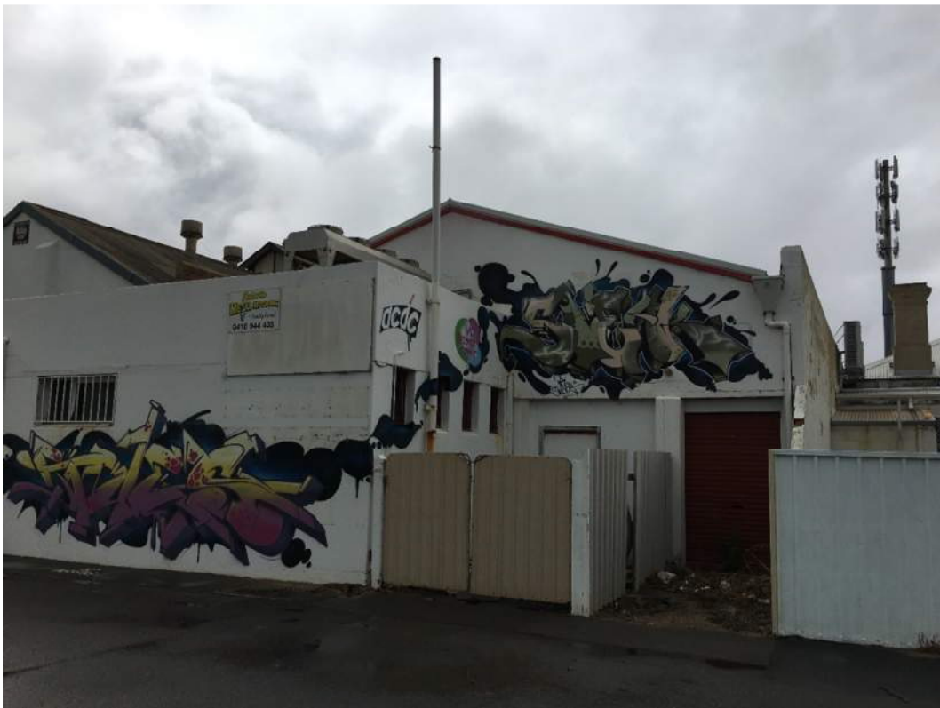
Figure 13: View of rear of building
