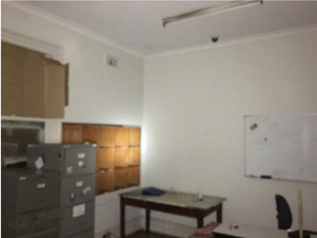
Figure 8: View of central space of building looking north
