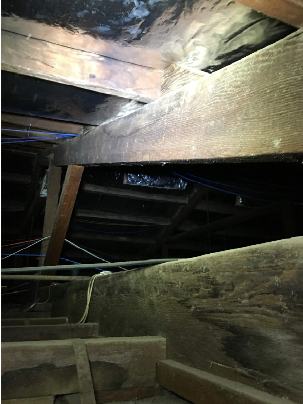
Figure 19: Close-up of Timber Truss
