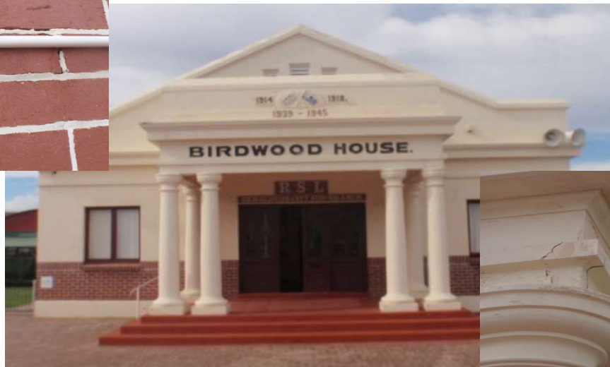
Birdwood House – requiring brickwork repointing and concrete cornice renewal
