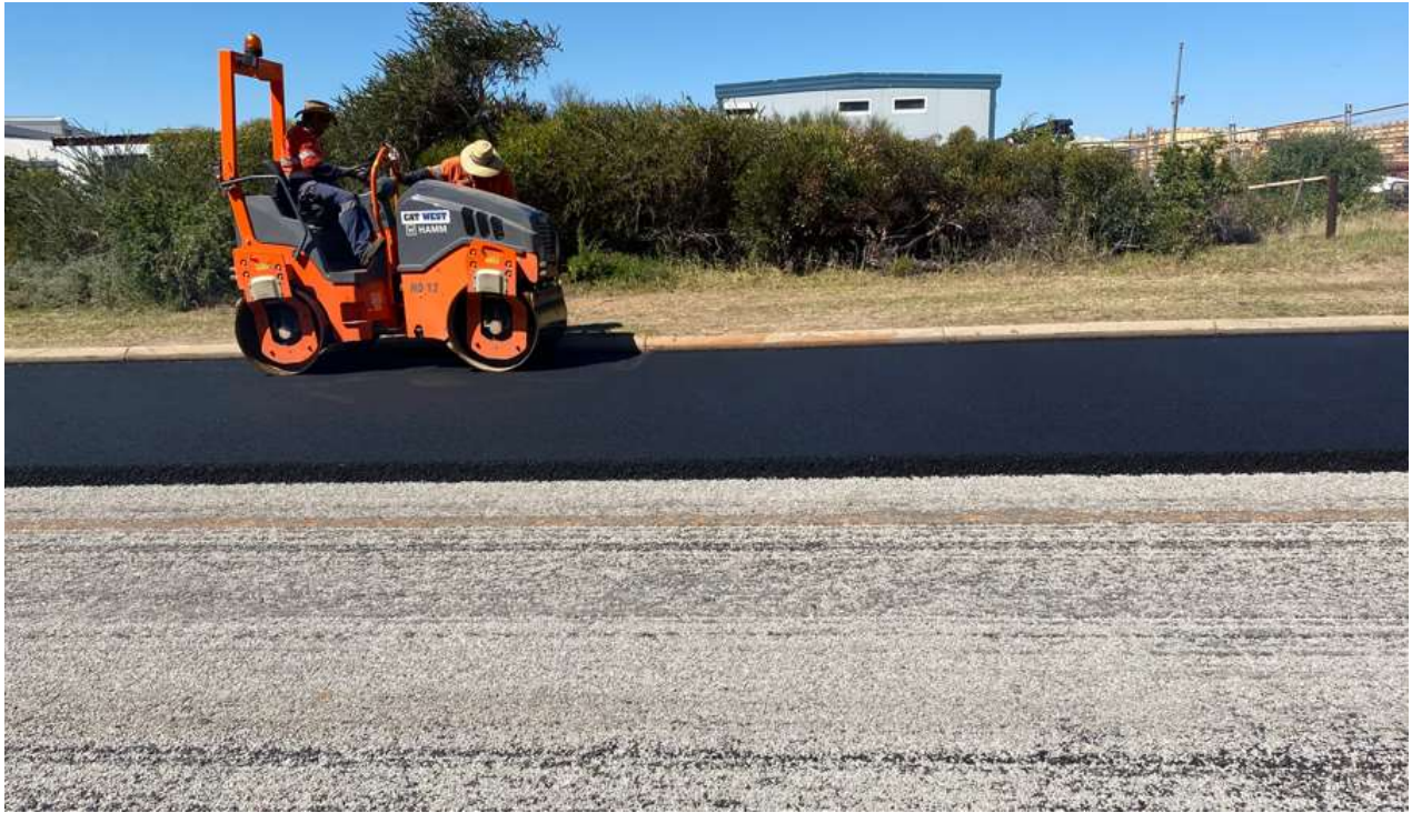
Example of resurfacing works - Point Street, West End 2022
