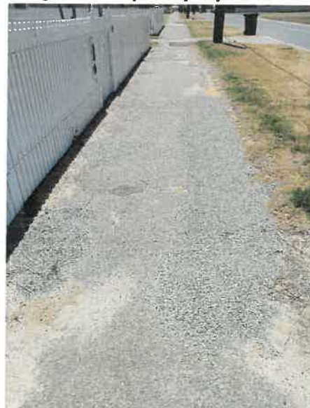
Image 4: Temporary repairs with loose blue metal
