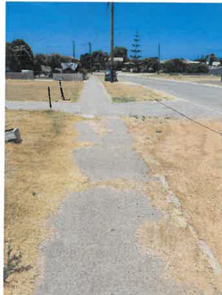
Image 1 and 2: The footpath is in disrepair, with cracks, rubble, weeds, and uneven surfaces.
