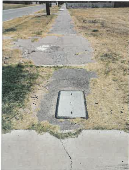
Image 1 and 2: The footpath is in disrepair, with cracks, rubble, weeds, and uneven surfaces.
