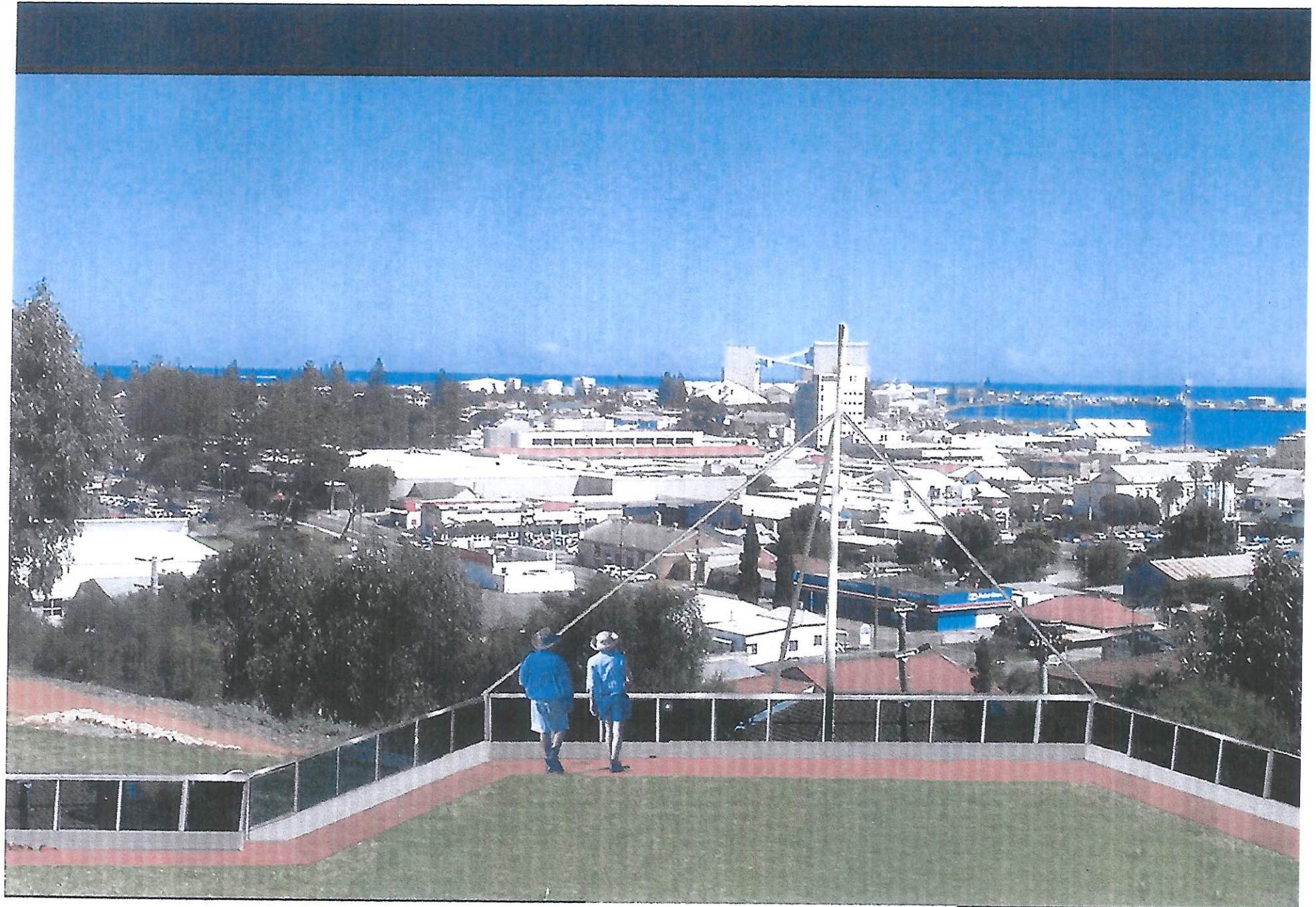
HMAS Sydney II Memorial Geraldton- "Sanctuary of the Deep"- Rest and Contemplation area Look Out Area - Roof of Sanctuary of The Deep
