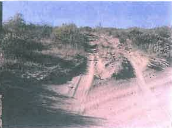
Unauthorised Access to High Vantage Point
