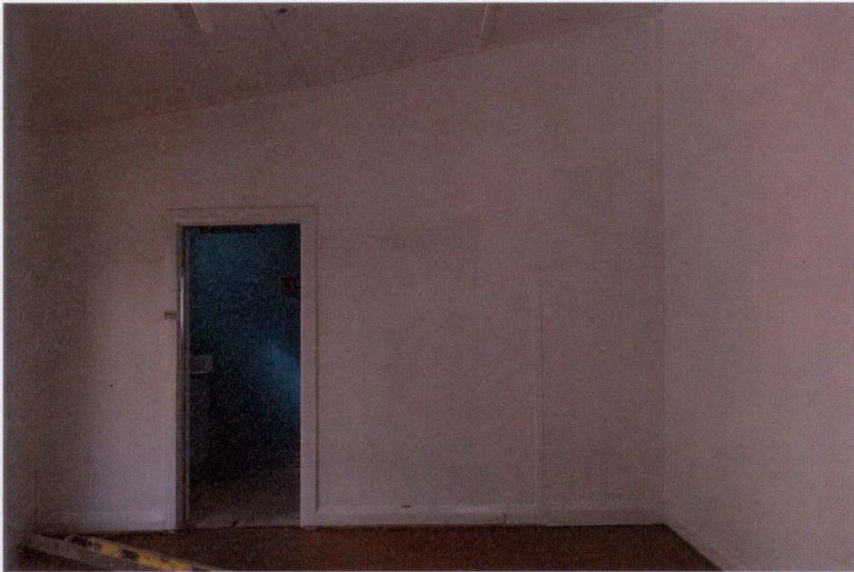
Infilled rear verandah looking south (Room 11) to the laundry.
