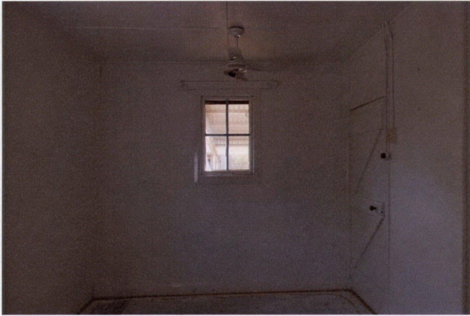
A combined bedroom and bathroom (Rooms 4 and 5). The line of the dividing wall can be seen in the floor.
