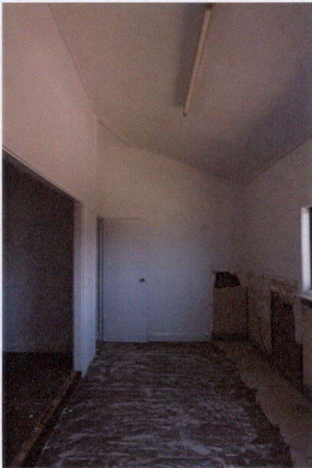
Eastern sleepout (Room 8) looking east.
