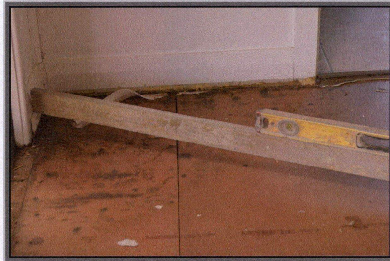
Plate 3 – Floor Subsidence
