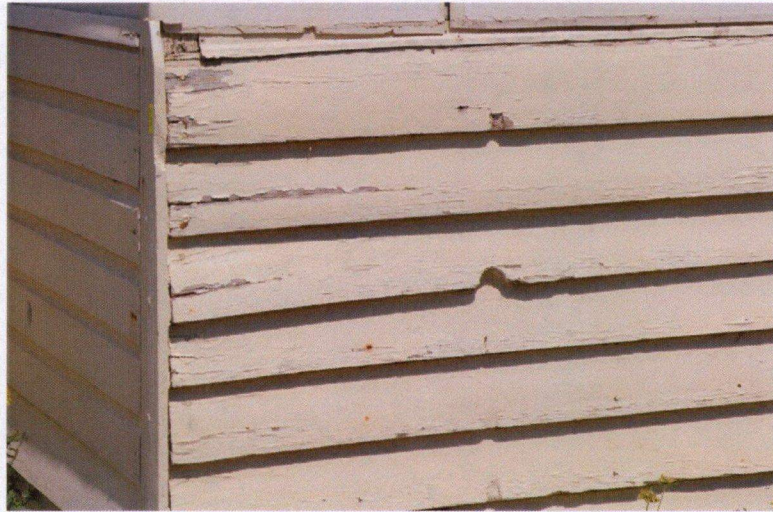
Plate 5 – Wall Cladding (weatherboard)
