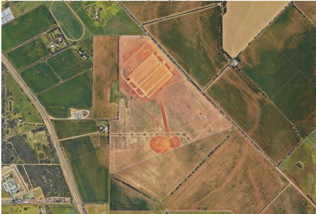
Figure 1: Aerial photograph of site during construction of existing facility
