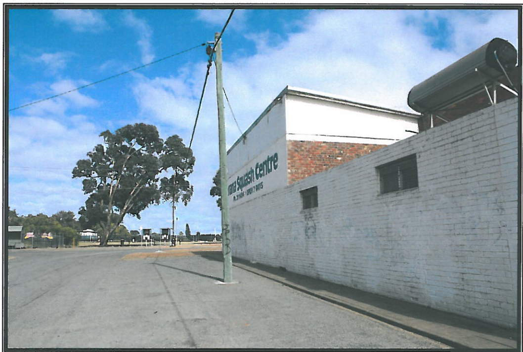
Carter Street (southern) elevation of development and parking
