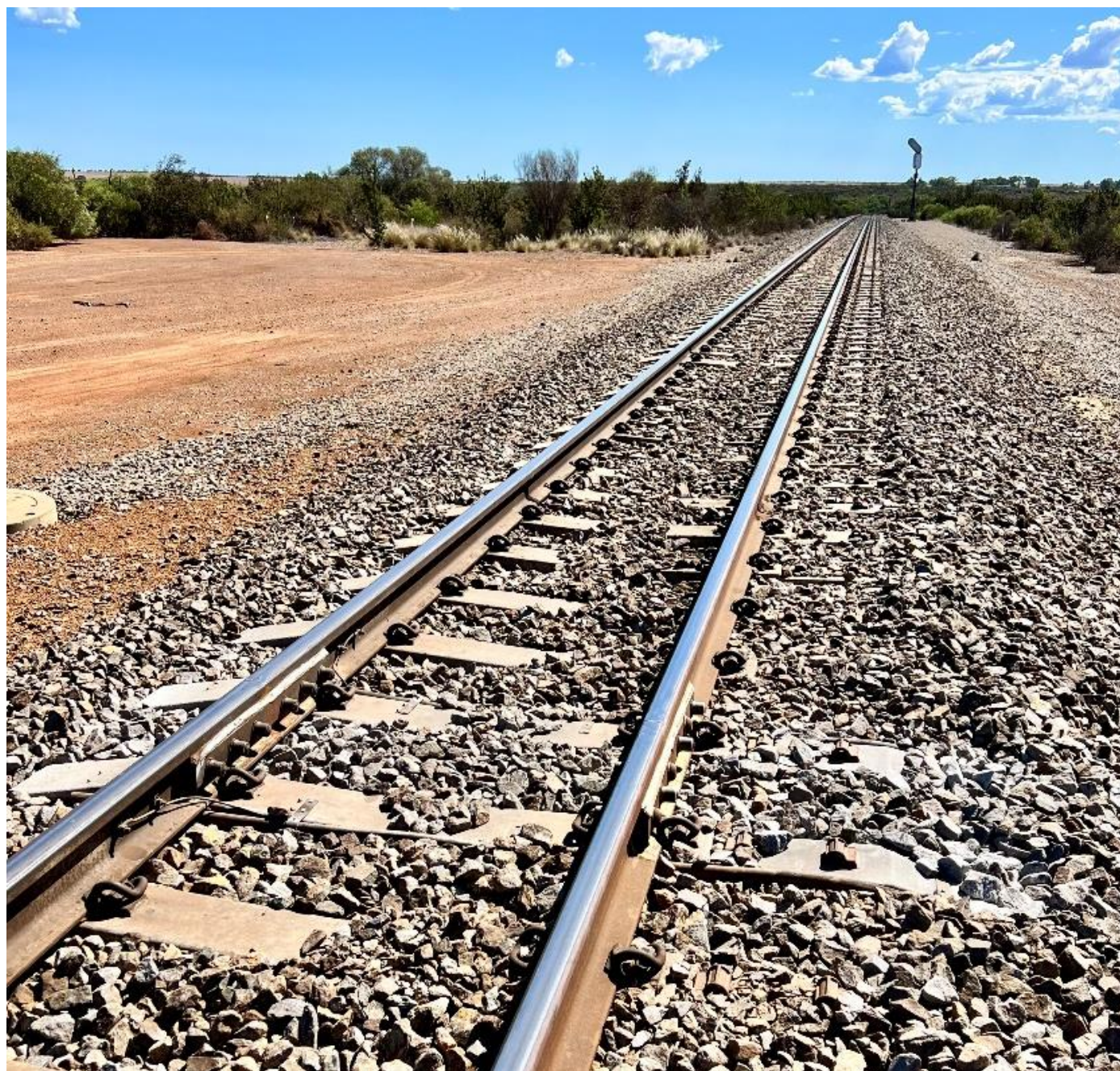
Figure 15 – Gauge Upgradable Concrete Sleepers (Geraldton-Mullewa Railway)
