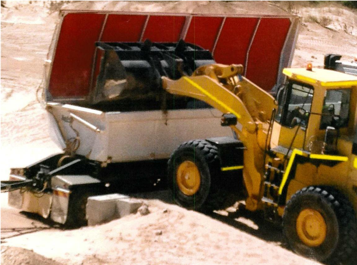
Figure 3.6 Loading Sand Directly into Waiting Road Trains (Mid West Sands)
