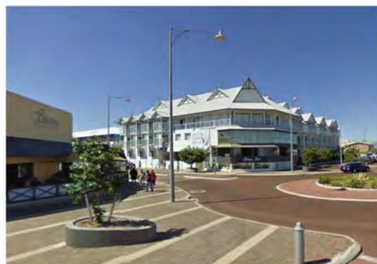
(Right) Example of land mark built form on corner street
