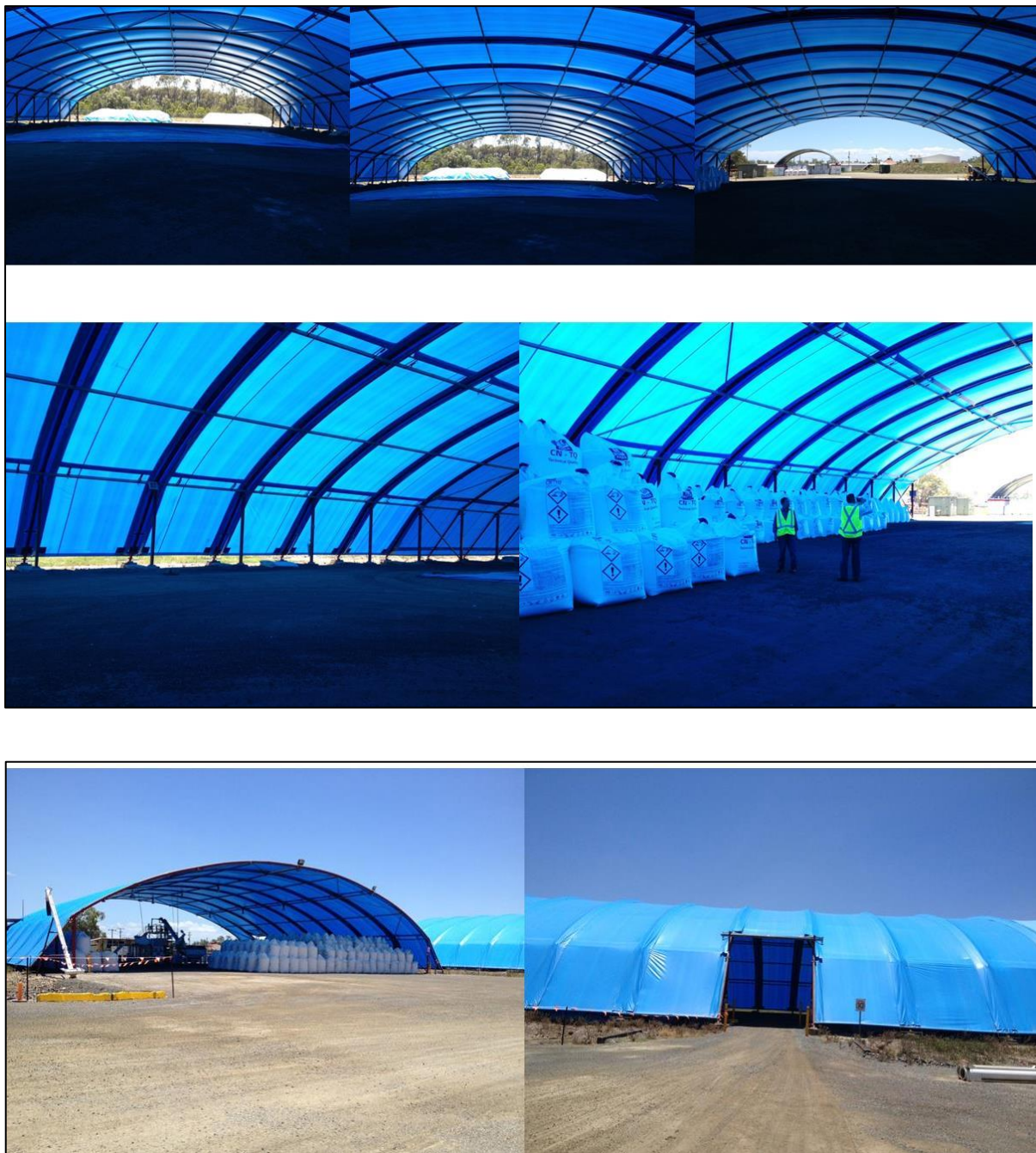
FIGURE 9 – ‘STATE OF THE ART’ FACILITY IN BAJOOL, QUEENSLAND
