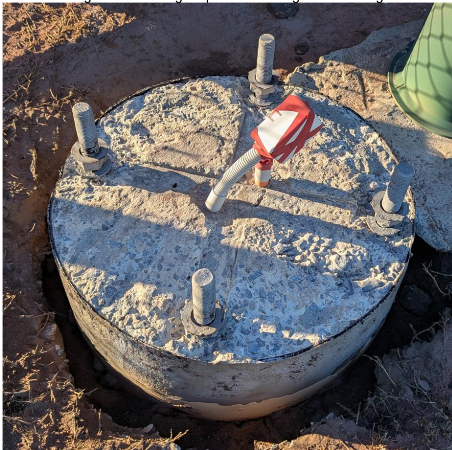
Figure 13: Footing for pole 3 following sand blasting.
