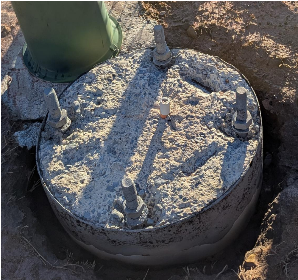
Figure 12: Footing for pole 2 following sand blasting.
