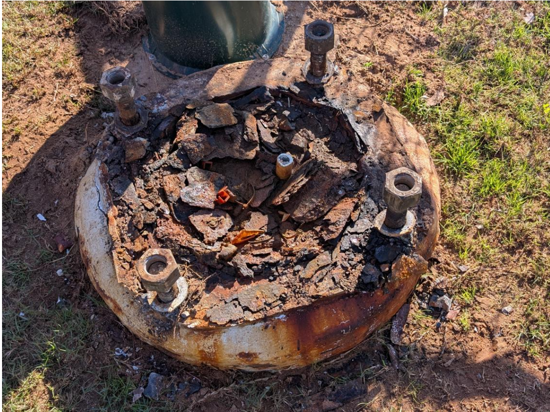
Figure 10: Light pole 2 footing.
