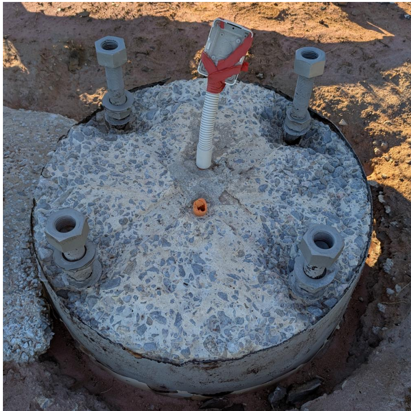
Figure 14: Footing for pole 4 following sand blasting.
