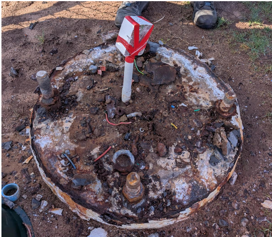
Figure 6: Light pole 3 Footing.
