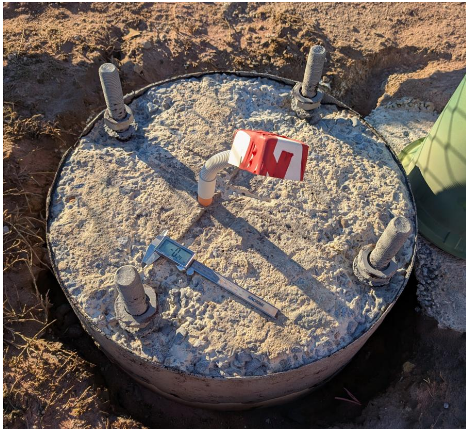
Figure 11: Footing for pole 1 following sand blasting.
