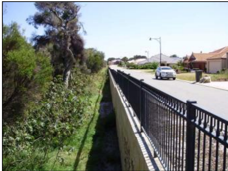
(Above) Example of 3m high retaining wall screened by vegetation
