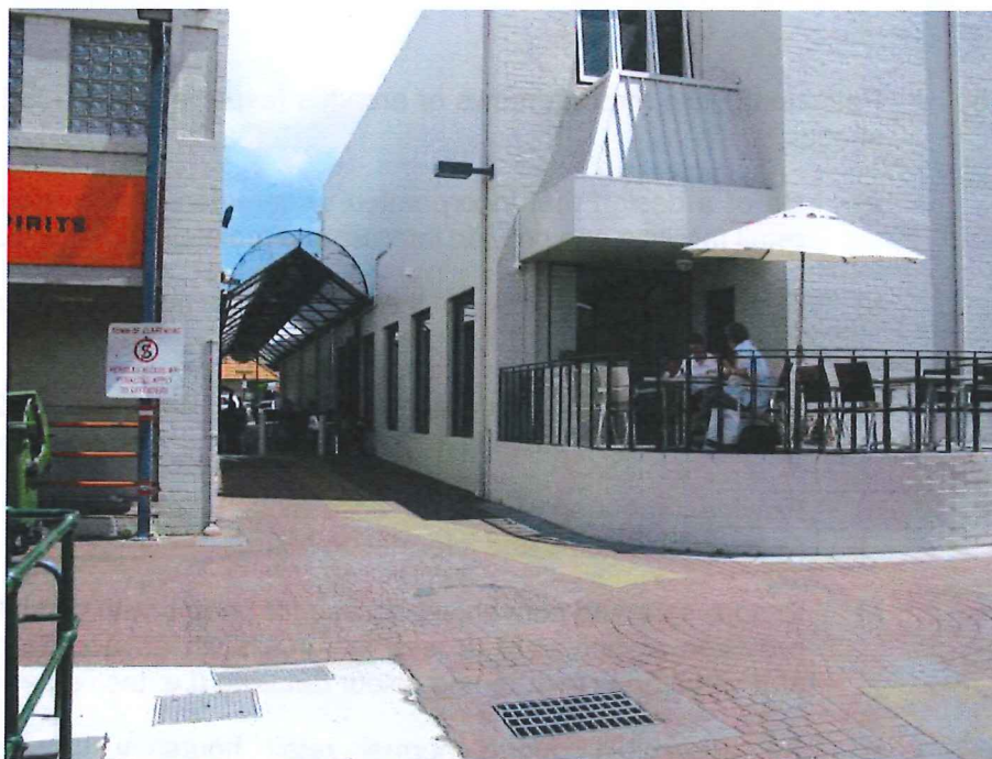
Figure 14 – An example of how to transform a service lane into a people lane (Lemon Lane, Perth – The former service lane has been partially covered and bollards installed to prevent vehicular traffic. The coffee shop has installed large windows along its side frontage to the former service lane to act as additional shopfront and to make the area visually larger and permeable. The covered area has alfresco dining and acts as a social place while still allowing pedestrian through traffic).
