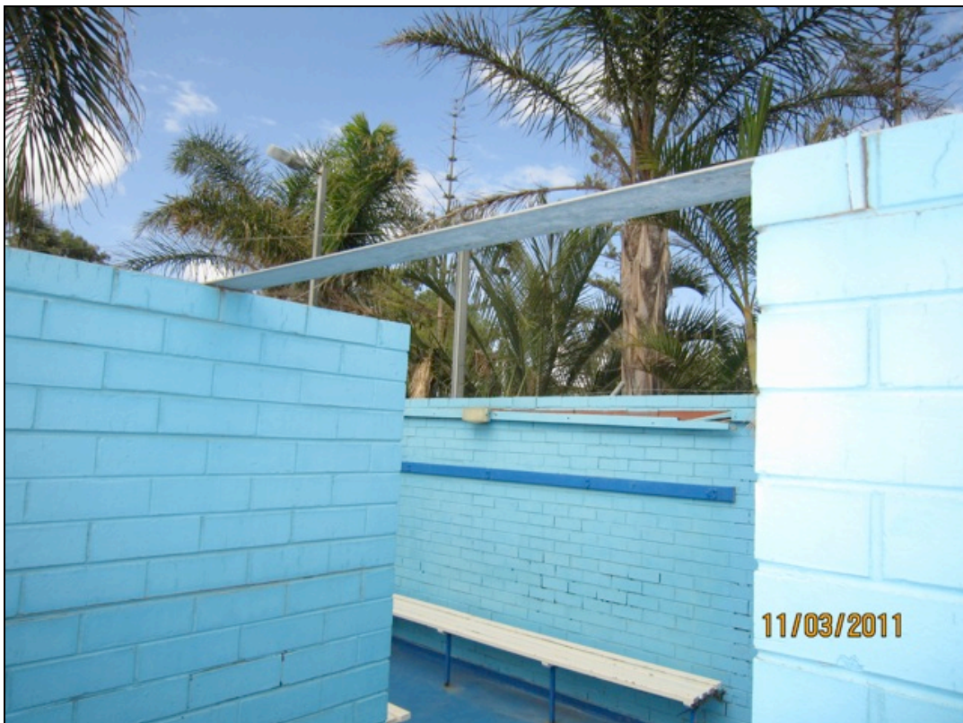
Photograph 2 - Steel flat bar installed to temporarily restrain brickwork
