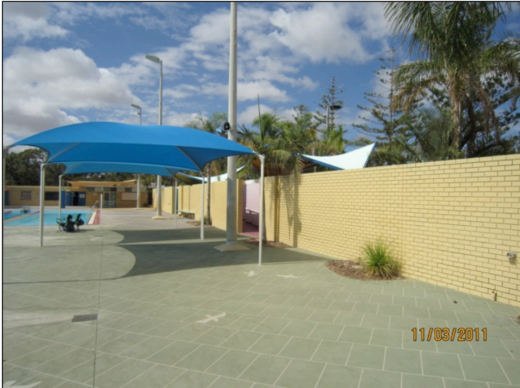
Photograph 1 - Outside wall of existing toilets/change rooms
