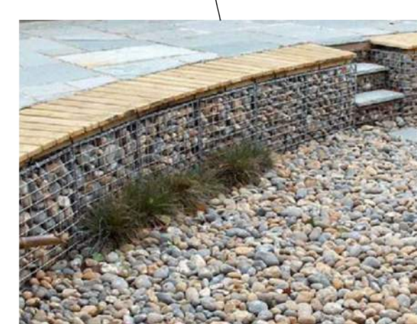
GABION SEATING WALLS - TYPICAL
