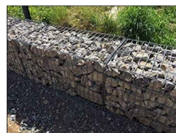
GABION DEFINITION OF FORMER HOUSES
