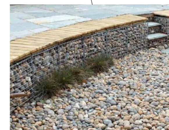
GABION SEATING WALLS - TYPICAL
