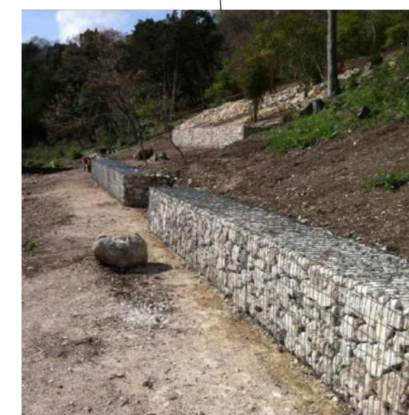
GABION RETAINING - TYPICAL
