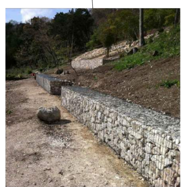
GABION RETAINING - TYPICAL
