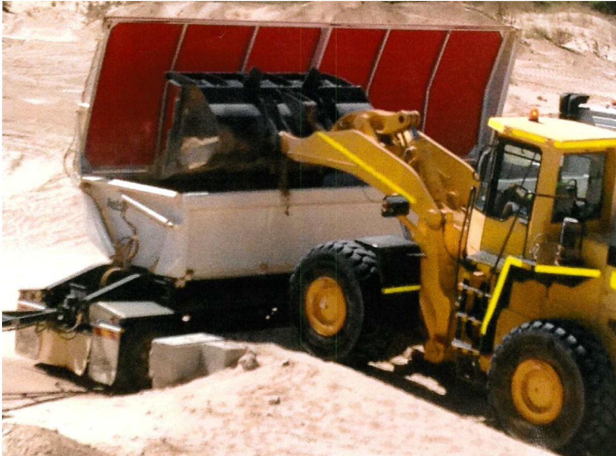
Figure 3.6 Loading Sand Directly into Waiting Road Trains
