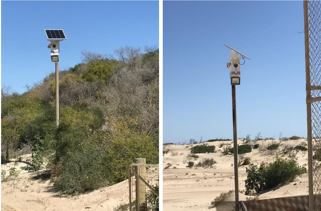
Figure 3.12 Surveillance at Compound Gate (Left) and Muster Point (Right)
