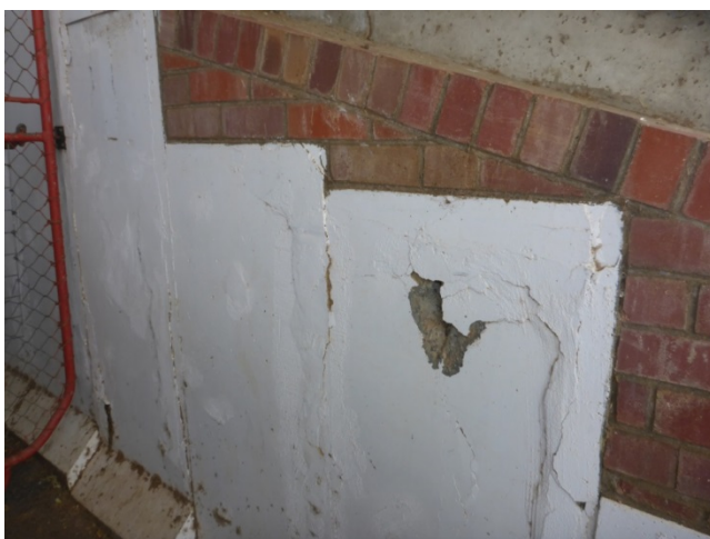
Pictures of spalling concrete in the Grand Stand tunnel
