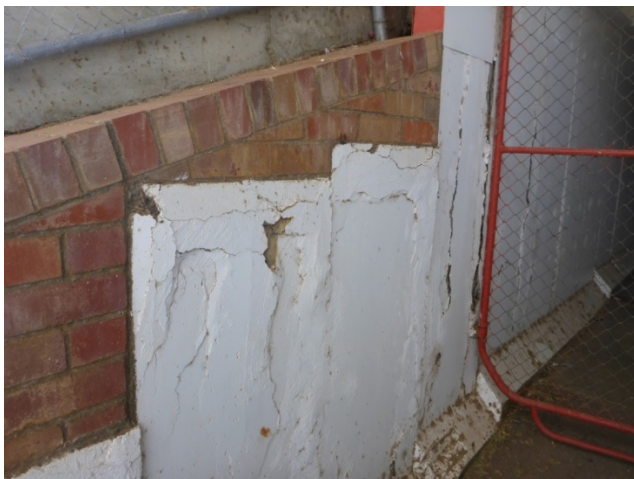
Pictures of spalling concrete in the Grand Stand tunnel
