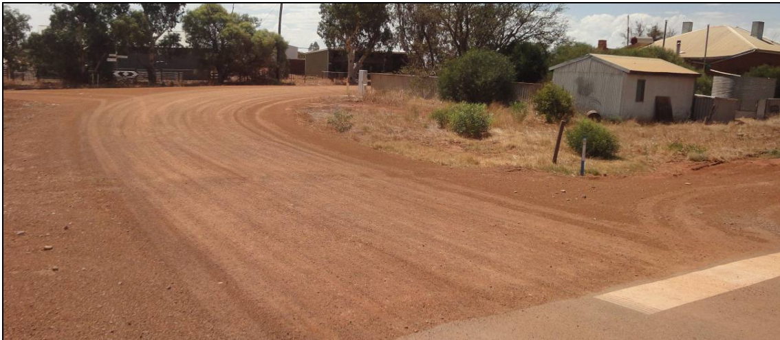
Fig 7.1 Northern approach to Eradu North Rd rail crossing
