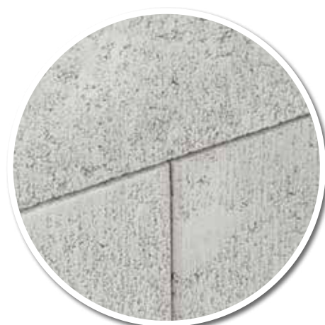
Clean wall with shadow lines
