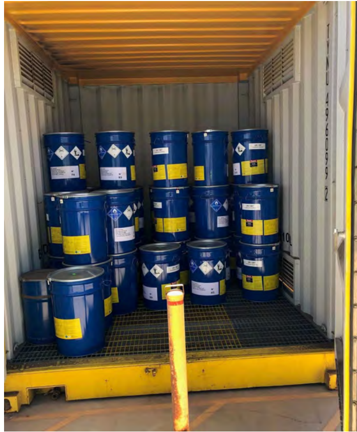
Photo 7 – *Inside Store PS2 showing ventilation and raised steel grating floor
