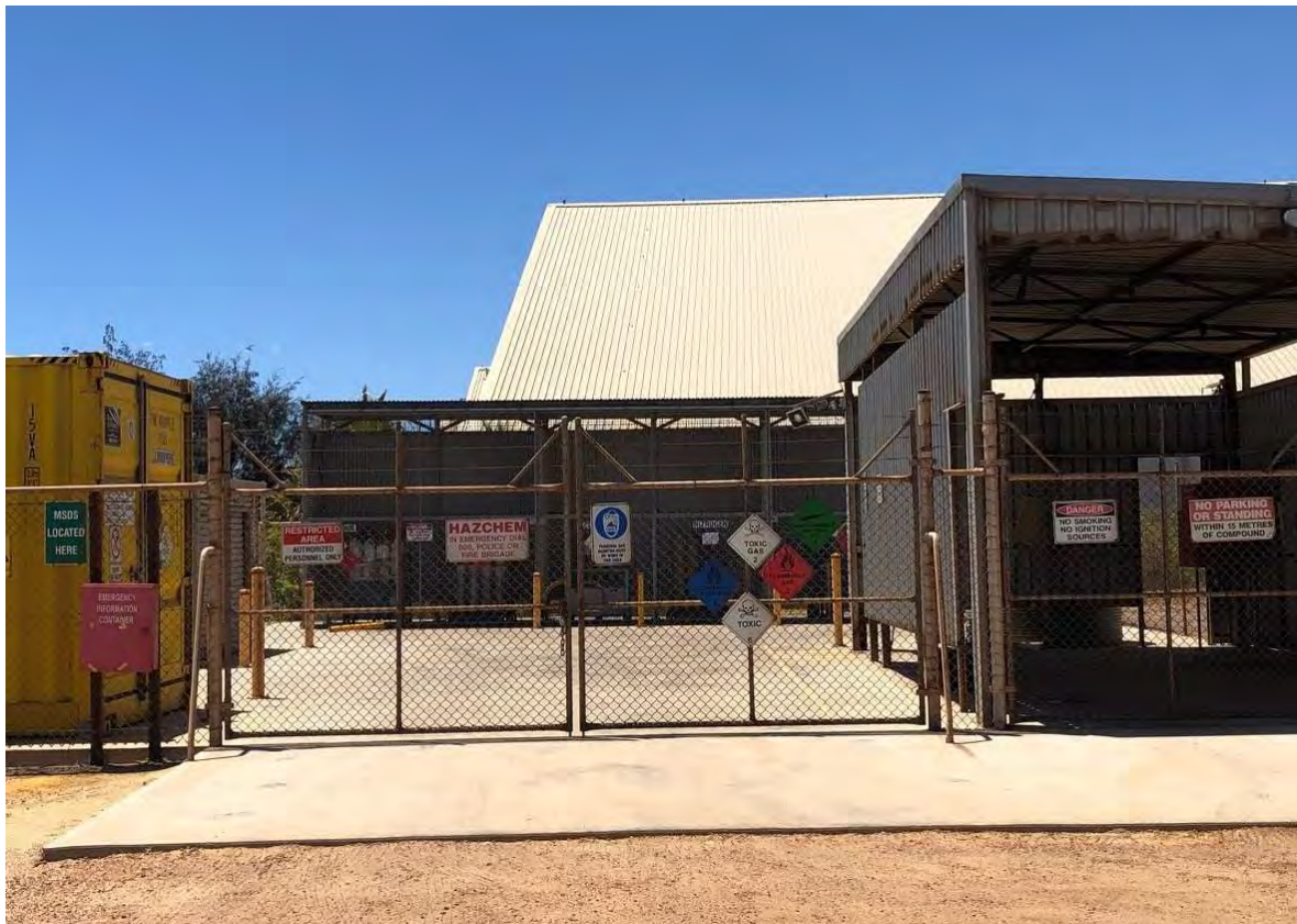
Photo 2 – *Front gates of the existing Geraldton DG compound showing warning signage and EIC
