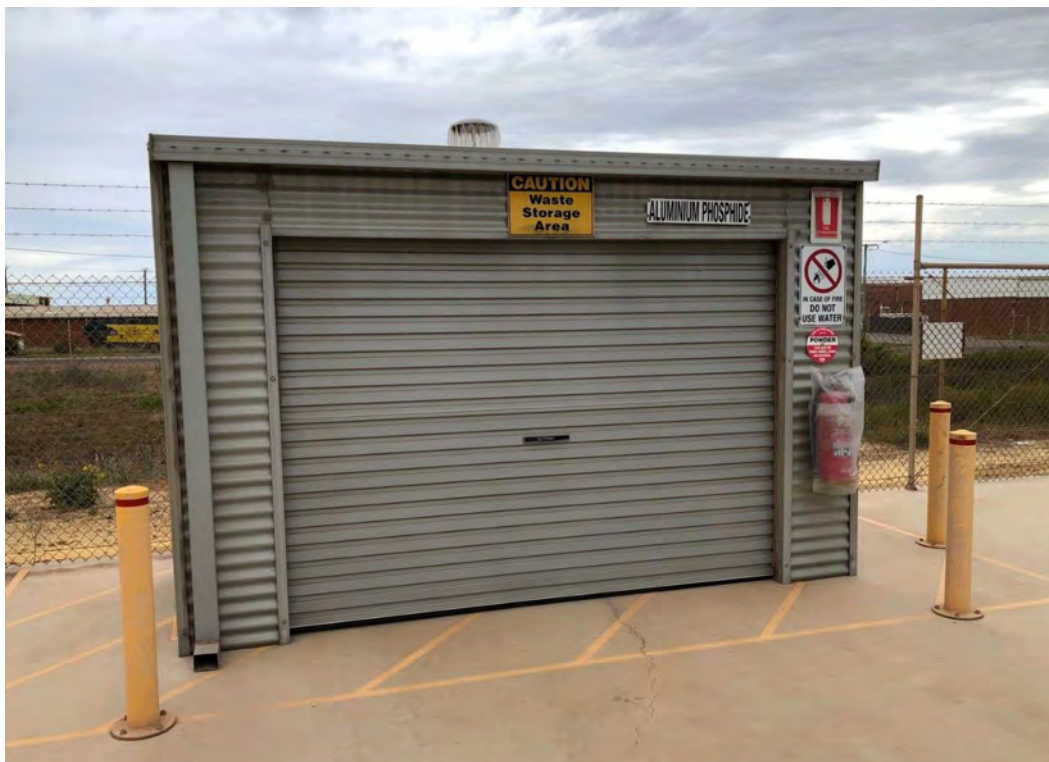
Photo 4 – *Locked AIP Waste Storage Area (Store PS3) showing gutter pipe, whirlybird vent, FEs, bollards and signage
