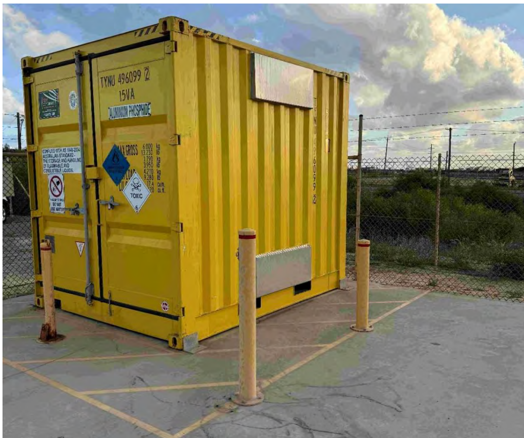
Photo 10 – *AIP Freight Container (Store PS2) showing signage, DG placards, bollards and covered vents
