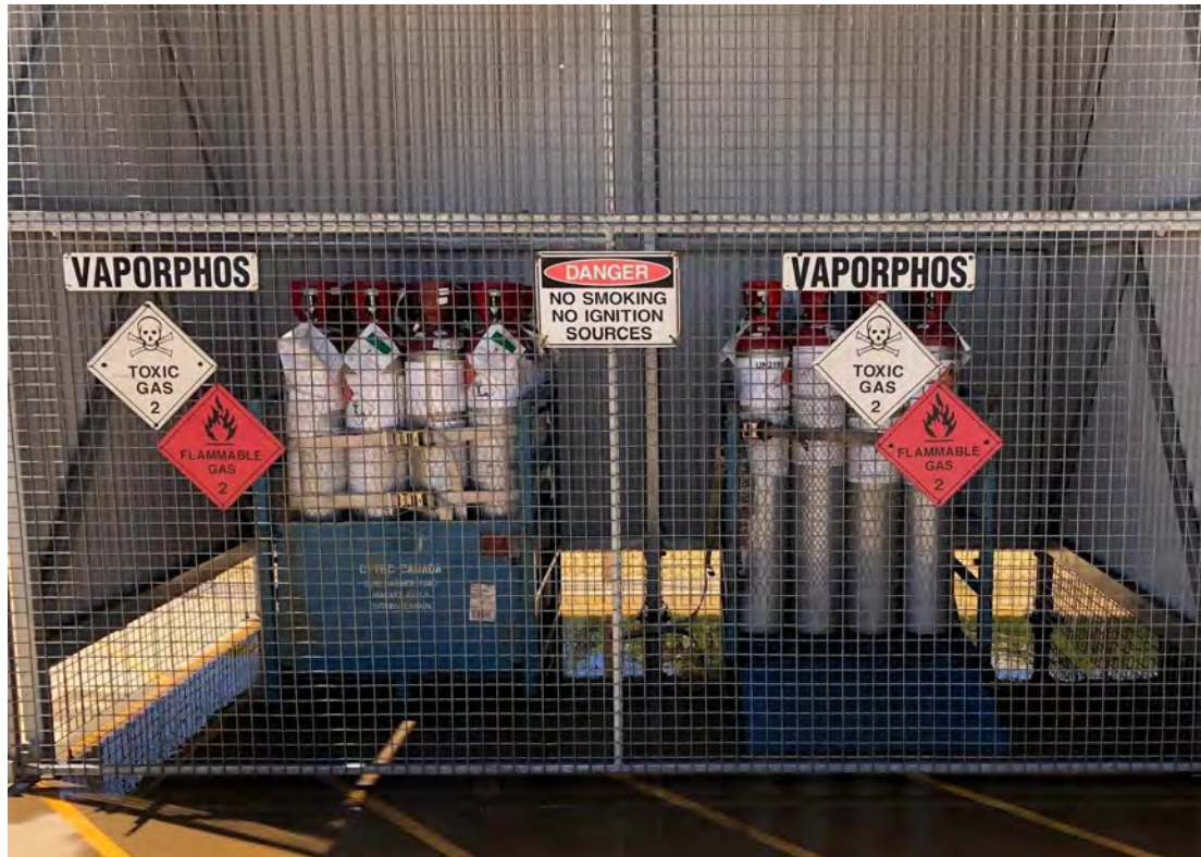
Photo 21 – *Store PS1 showing DG placarding / signage and stillages of VaporPhos cylinders
