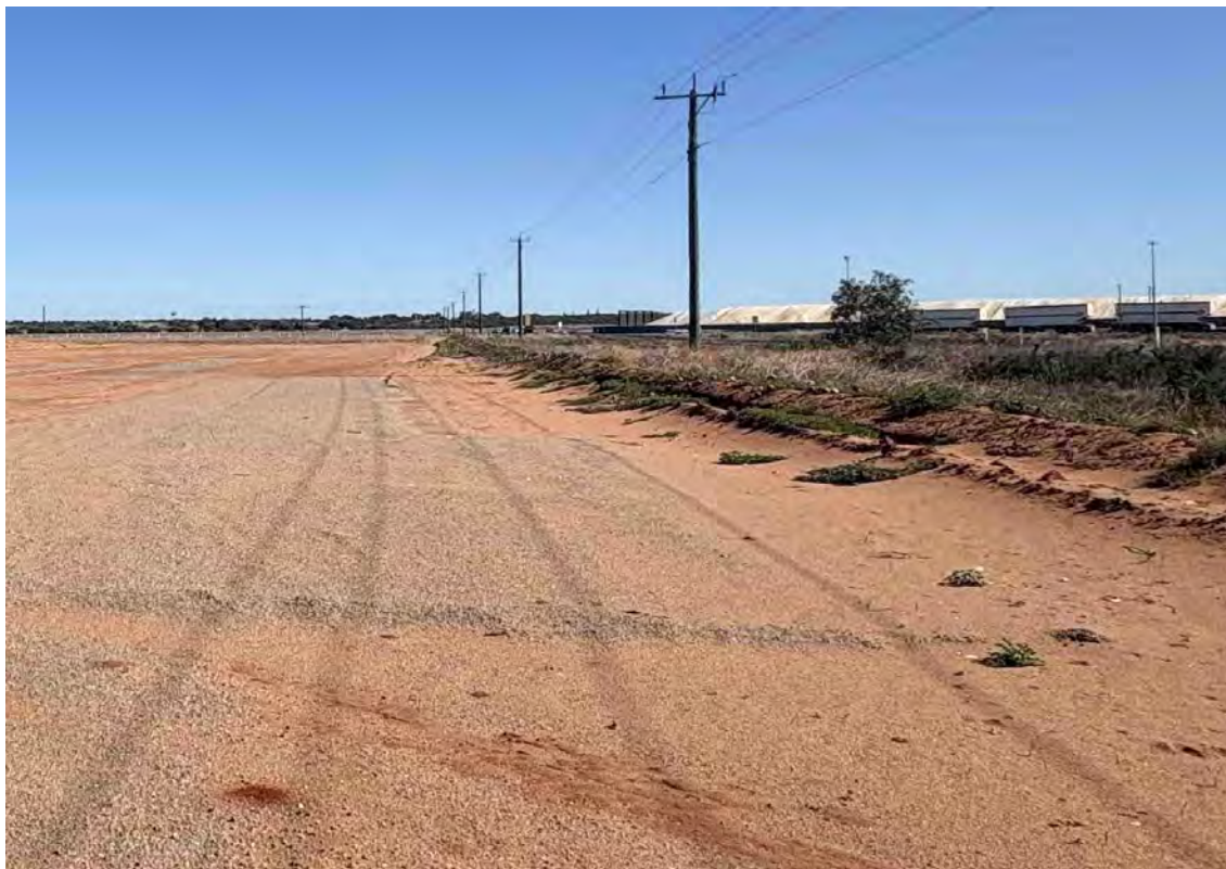
Photo 30 – Proposed location of the Narngulu DG compound showing lighting at weighbridges
