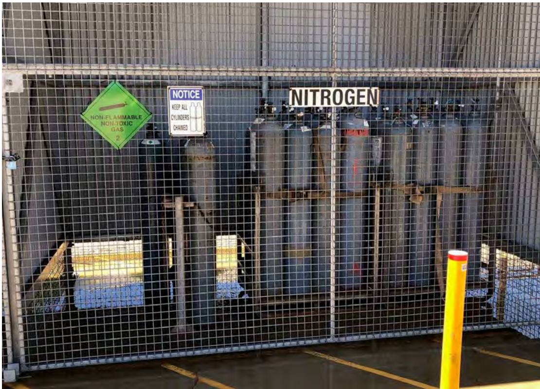
Photo 23 – *Store PS1 showing signage, DG placarding and restrained cylinders of Nitrogen
