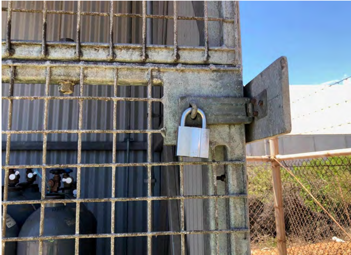
Photo 5 – *Gas Cylinder Store (Store PS1) showing locked front gates
