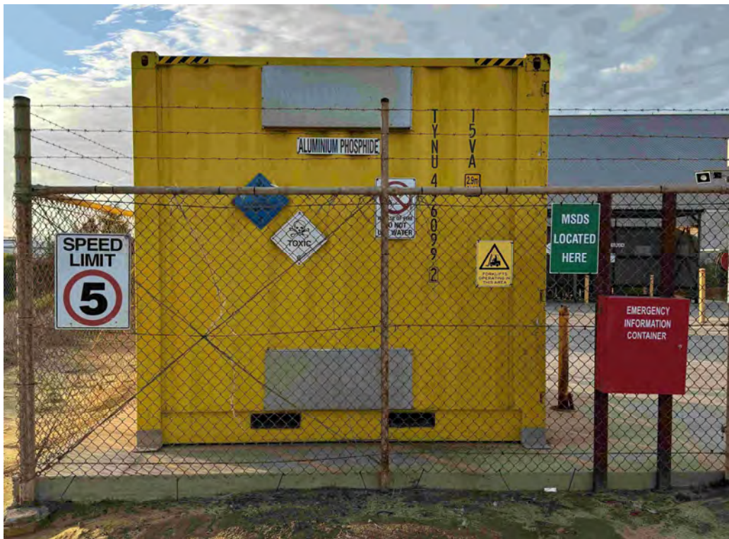
Photo 18 – *DG placarding and signage on the side of Store PS2 and EIC
