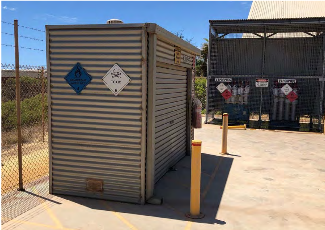
Photo 19 – *FE, DG placarding and signage on the AIP Waste Storage Area (Store PS3)
