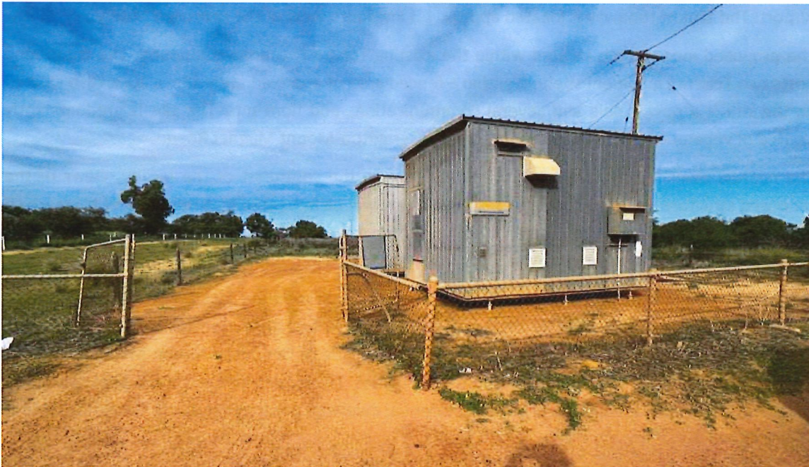
FIGURE 2 SITE ENTRY AND EXISTING EXCHANGE EQUIPMENT BUILDINGS
