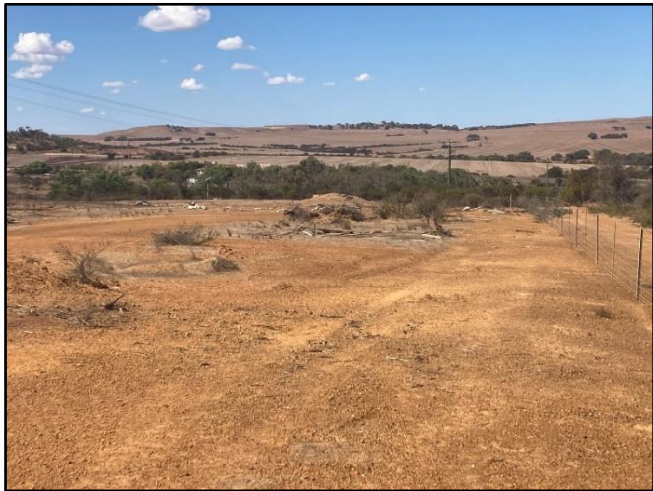
Photo 2: Area where material will be tipped from truck and then loader used to move material to stockpile location
