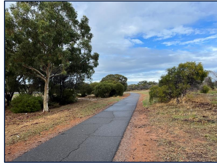
Figure 5 Existing dual use path on eastern boundary
