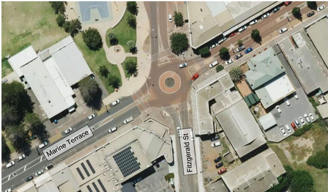
Figure 2-4 Marine Terrace / Fitzgerald Street Intersection
