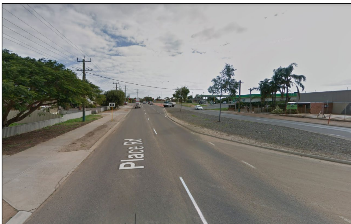
Figure 4: Westbound view along Place Road
