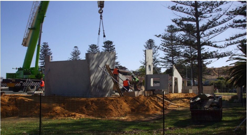
QEII extensions 19 November 2007. Erection of the tilt panels.
