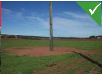
Power pole cleared 3 metres around base.
