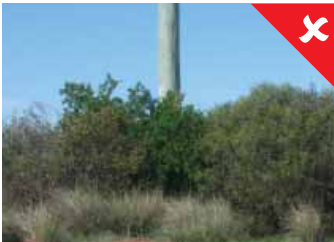
Power pole not cleared from flammable material.
