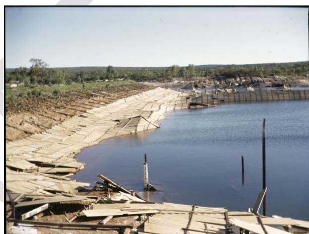
View of collapsed roof, 1968. Courtesy SLWA image b4569262_1
