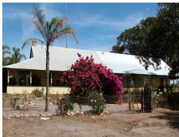
Municipal Heritage Inventory 2005. Façade of House.
