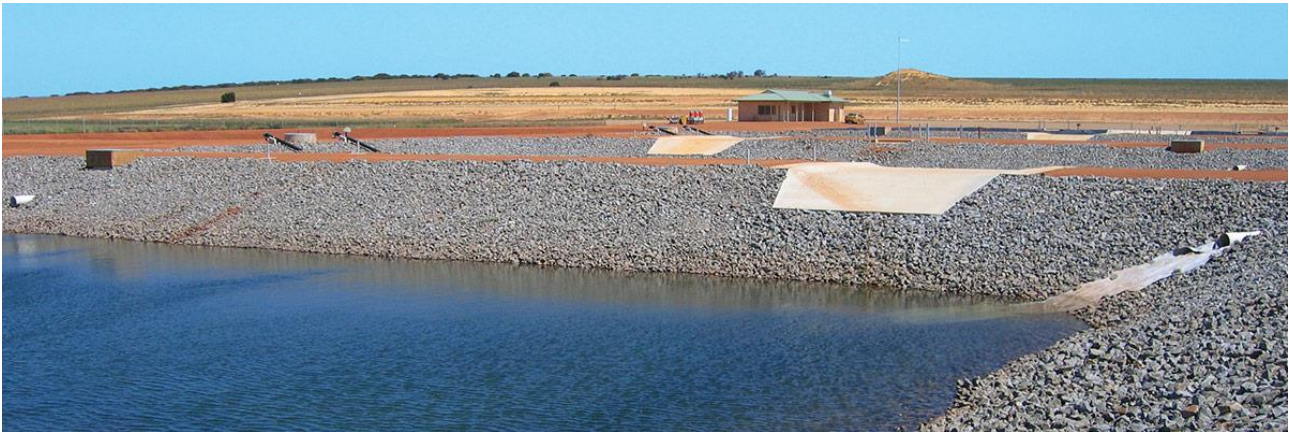
Figure 6-3 Narngulu Wastewater Treatment Plant (Source: DM Civil)
