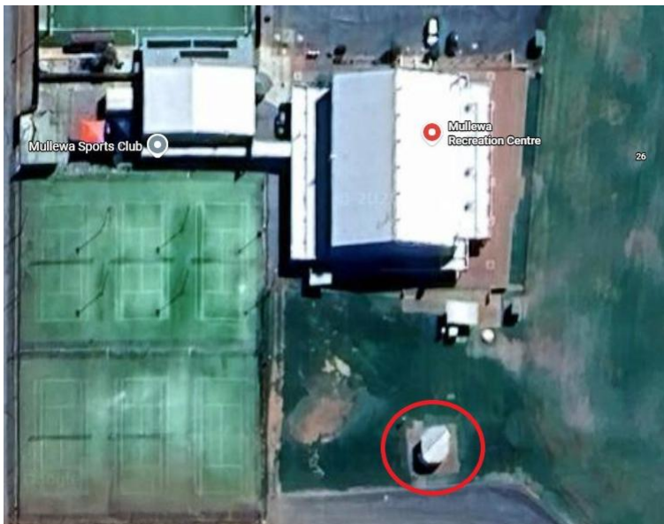
Image 2 – Aerial view of ablution block
