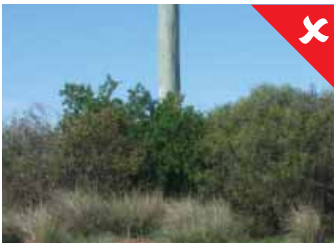
Power pole not cleared from flammable material.
