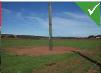
Power pole cleared 3 metres around base.
