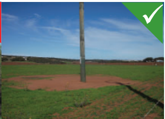
Power pole cleared 3 metres around base.
