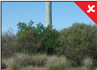
Power pole not cleared from flammable material.
