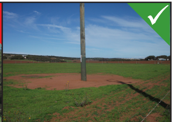
Power pole cleared 3 metres around base.
